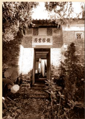
鏡蓉書屋修葺前的外貌 The main entrance of the Kang Yung Study Hall before restoration
