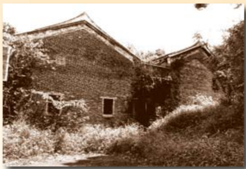
修復前的山牆 Gable walls of the building before restoration
