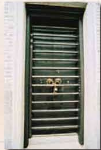
傳統木柵拉門 Traditional sliding timber grille door
