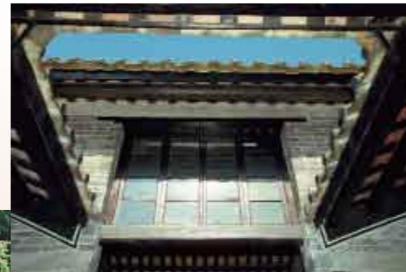
古屋主要依靠天井採光和增加室內空氣流通 The interior of the house relies on the courtyard for daylighting and ventilation
