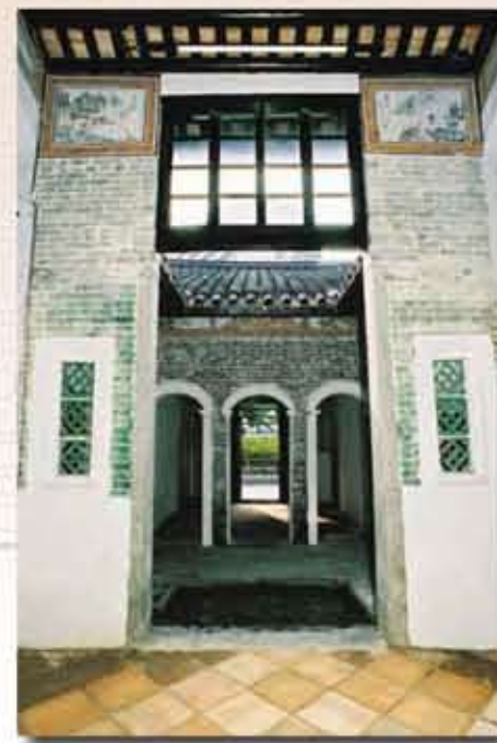
古屋內部的地面鋪設菱形圖案的廣東大階磚 The floor inside the Old House is paved with Canton tiles in diamond patterns
