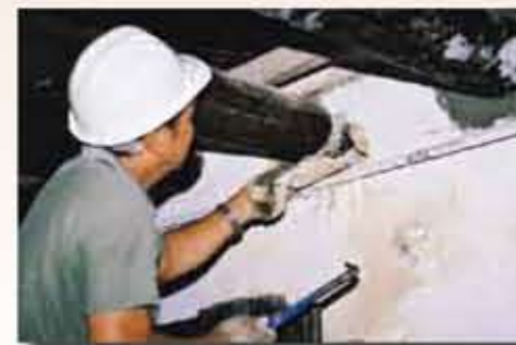
更換損毀的樑條 Replacement of defective purlin
