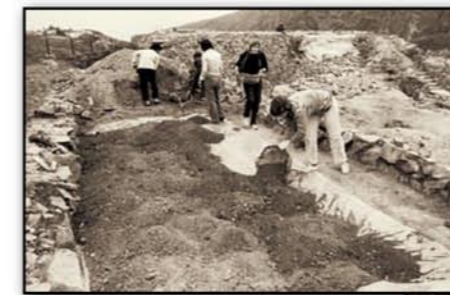
修葺東牆的平台 Repairing the platform of east wall
