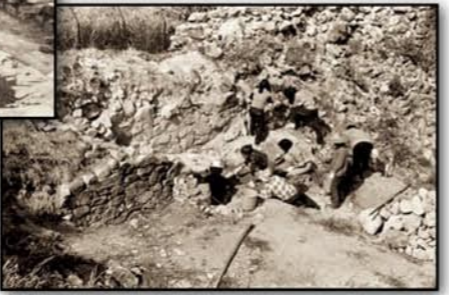
修復倒塌的城牆 Restoring the collapsed wall
