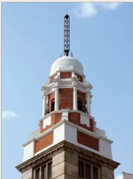
鐘樓頂部的混凝土圓拱頂及避雷針 Top of the Clock Tower with concrete dome and lightning rod
