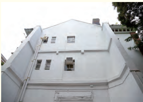
一九六六年發生嚴重山泥傾瀉後，倒塌部分加建兩道扶壁。 Two buttresses were erected at the collapsed portion after the severe landslide in 1966.
