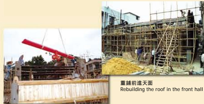
安裝主樑 Installation of the main beam
