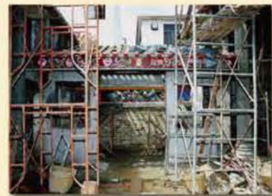
女兒牆已安放在廂房的牆壁內供人觀賞 The parapet was installed on the wall of the side room for display
