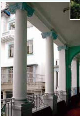
北座遊廊的石柱 Stone columns of verandah of the North Block
