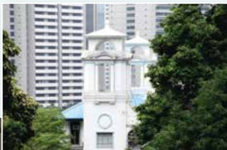
北座屋頂的塔樓 Towers on the roof of North Block
