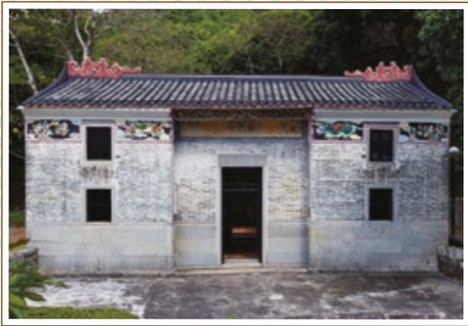
古屋正立面 The facade of the Old House
