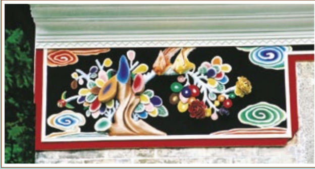
建築物正面精巧的灰塑 Decorative mouldings on the facade of the house
