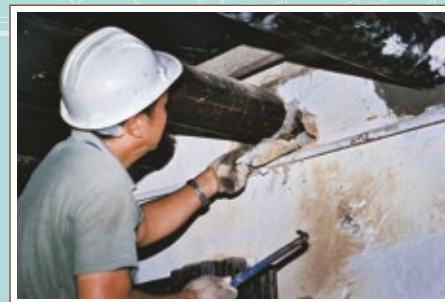
更換損毀的樑條 Replacement of defective purlin
