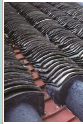
天面以客家式瓦片覆蓋 The roofs are covered with Hakka-style tiles
