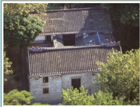
古屋為傳統客家的兩進一天井三開間式建築 The Old House is a typical traditional Hakka residence having a layout of two-hall-one-courtyard with three bays.
