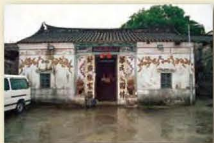
張氏宗祠修復前的外貌 The Cheung Ancestral Hall before restoration
