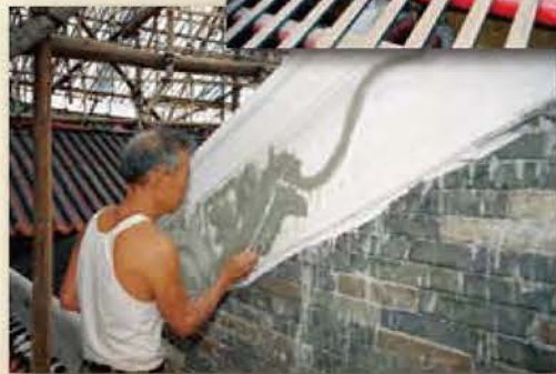
工匠於牆頭上重新飾上灰塑 Redecoration of plaster mouldings on wall frieze
