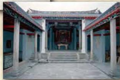
修復後的天井及正廳 The restored courtyard and main hall
