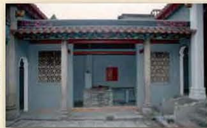
天井廂房的廚房 Kitchen at the chamber of the courtyard
