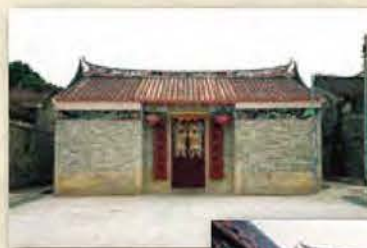
修復後的外貌 The restored façade of the building
