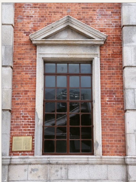
鐘樓的長方形玻璃窗，配以木框、花崗岩窗框和三角形楣飾。 The rectangular glass window on the Clock Tower has wooden-frame, granite window surrounds and pediment window head.
