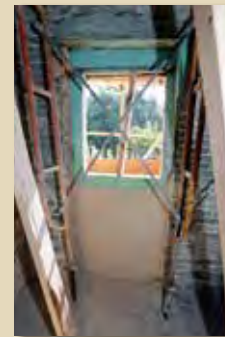
修復期間展露出一樓窗戶的原有門洞痕跡 Remnants of the original door at a window on the first floor were revealed during restoration
