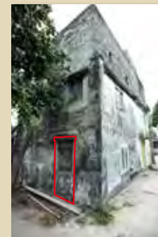
修復前地下側門曾改作窗戶 The side door on ground floor had been converted to a window before restoration
