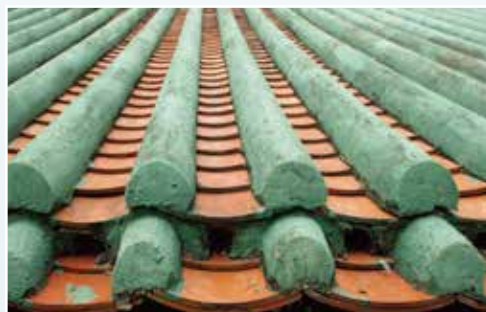
以中式柏油瓦鋪蓋的斜形屋頂 Pitched tarred Chinese tiled roof
