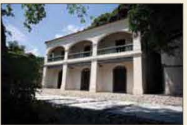
修復後的外貌 The building after restoration
