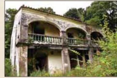
修復前的外觀 The building before restoration
