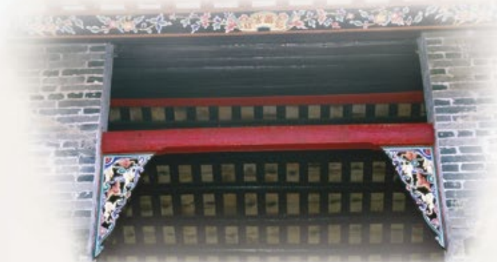
樑下雕有蝠鼠的雀替 Decorative joint brackets with bat carving patterns under the beam
