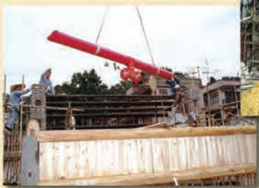
安裝主樑 Installation of the main beam
