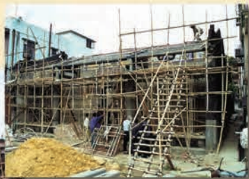
重鋪前進天面 Rebuilding the roof in the front hall
