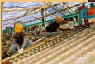
工人正在鋪砌前進天面瓦頂 Workers laying roof tiles at the front hall
