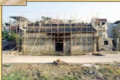
復修工程進行中 Restoration work in progress
