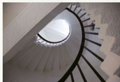
燈塔內石砌的螺旋式樓梯 Masonry circular staircase in the lighthouse
