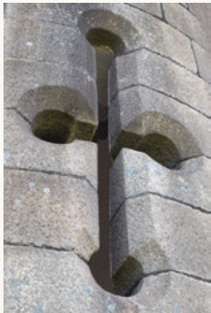
舊青洲燈塔牆上的「十」字開口 Cross-shaped opening on the wall of the old Green Island Lighthouse
