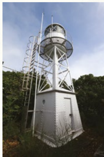
燈籠洲燈塔的外貌 Exterior of Tang Lung Chau Lighthouse
