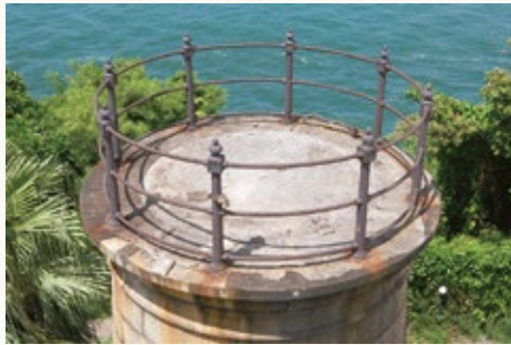
舊青洲燈塔頂部 Roof of the old Green Island Lighthouse
