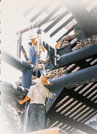
一九九四年工人正在 修復中進的天面結構 Workers restoring the roof structure of the middle hall in 1994
