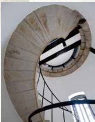
新青洲燈塔內以磚石鋪砌的螺旋形樓梯 Spiral staircase made of fine masonry in the new Green Island Lighthouse
