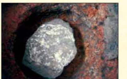
小坑村明代柱洞遺蹟及石上六角形立柱的痕蹟 Trace of hexagonal column on the foundation stone in a Ming dynasty posthole, Siu Hang Tsuen
