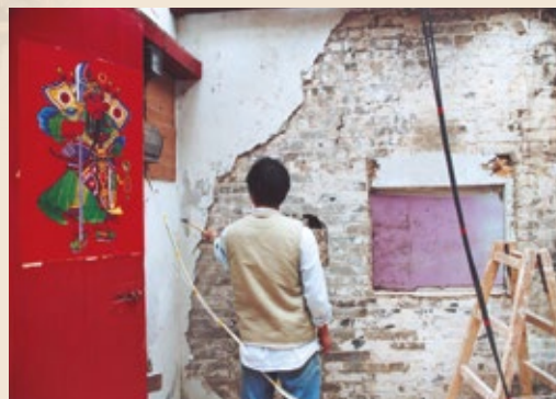
工人正在鑿去牆身的批盪 Removal of the rendering to expose the original brickwork
