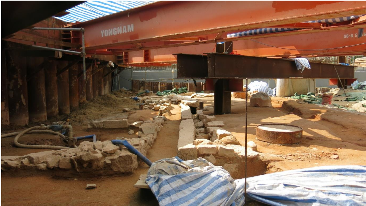
Photo E1 T1 tidied up before backfilling
