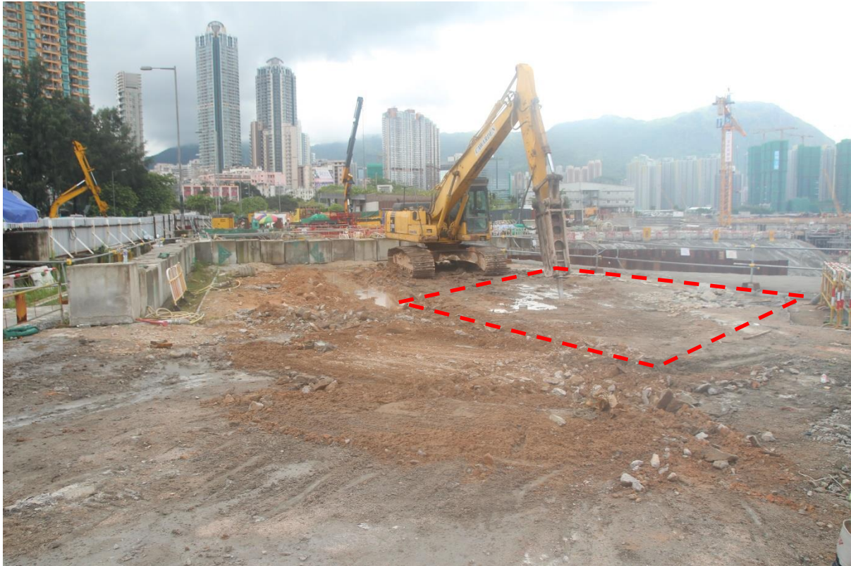
Photo C1 Location of KSWT2016 Trench 1
