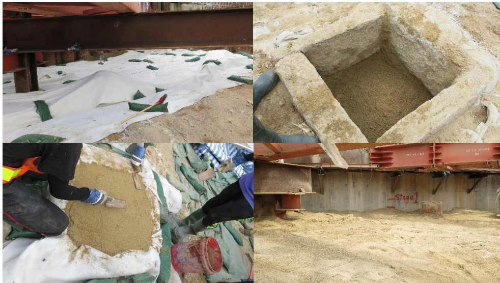
Photo E2 Features covered with water-permeable canvas, J1 backfilled with sands and stabilized with sand bags and covered, the whole T1 filled with 500mm sand
