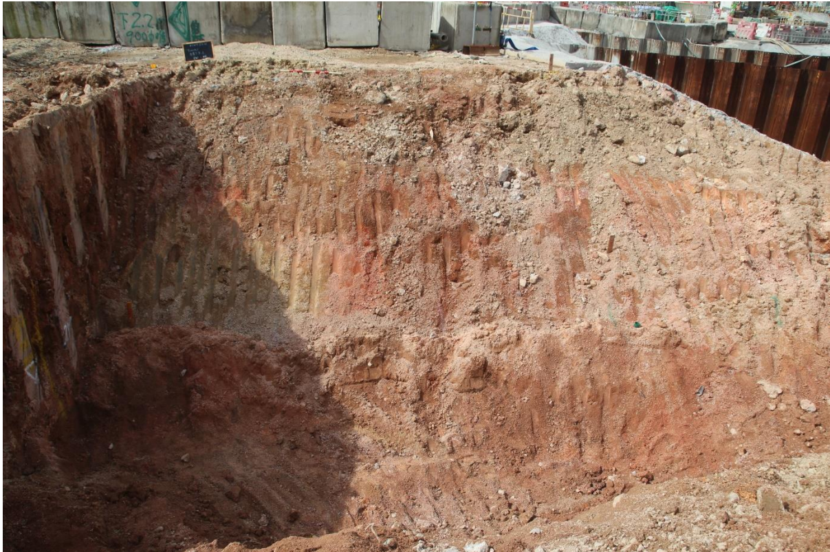
Photo C5 Excavation of KSWT2016 Trench 1 (SW to NE)
