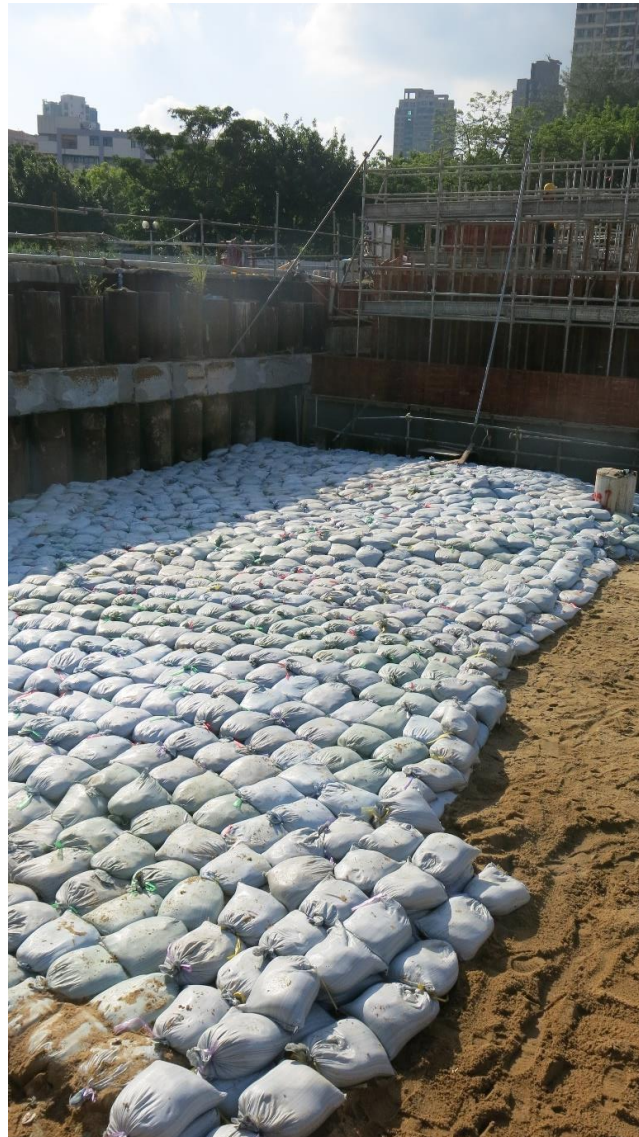
Photo E4 Covered the T1 with 2 layers of sand bags
