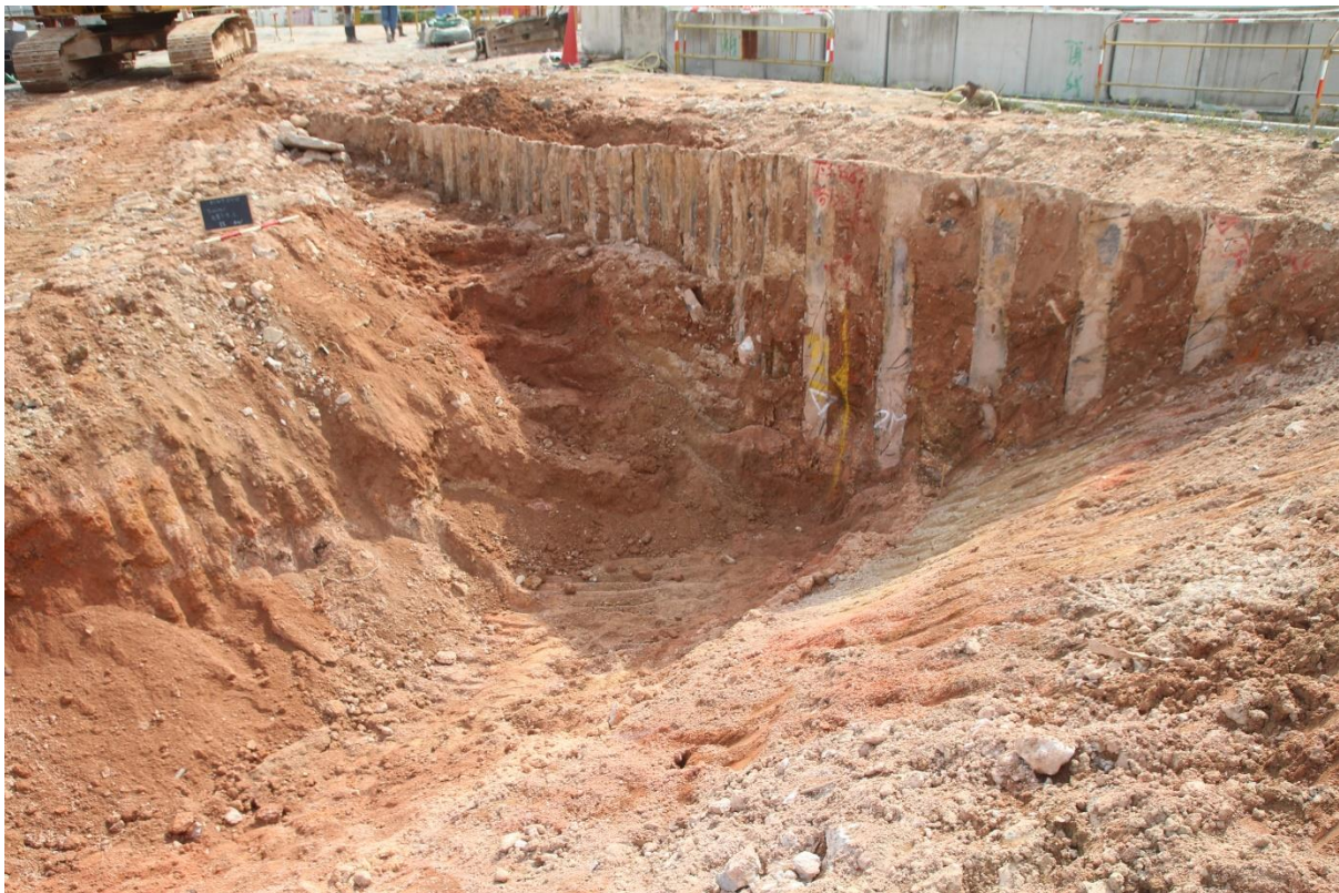
Photo C4 Excavation of KSWT2016 Trench 1 (SE to NW)
