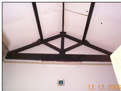
Exposed timber roof truss at the west end room
