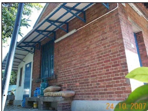
Later added canopy at west elevation
