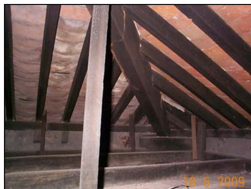
Soffit of the roof from the access panel at the false ceiling of the 1/f verandah – the hip ridge at the corner of the roof
