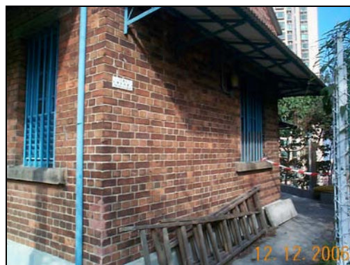
Later added canopy at east elevation
