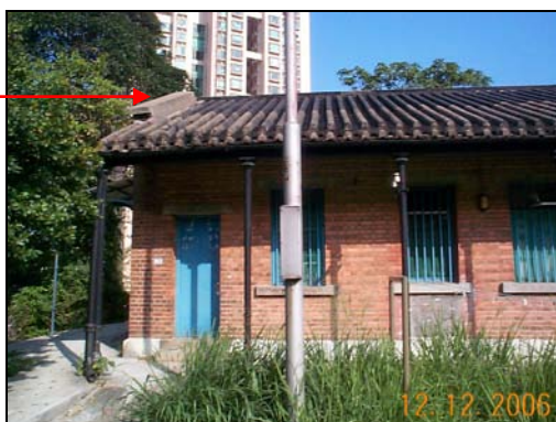
Granite coping on top of west gable wall
