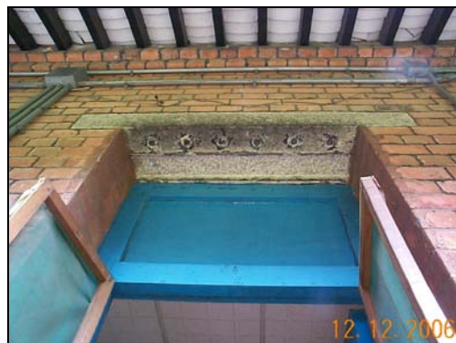
Original window changed to door shown by the holes in the granite lintol after removal of the iron vertical security bars
