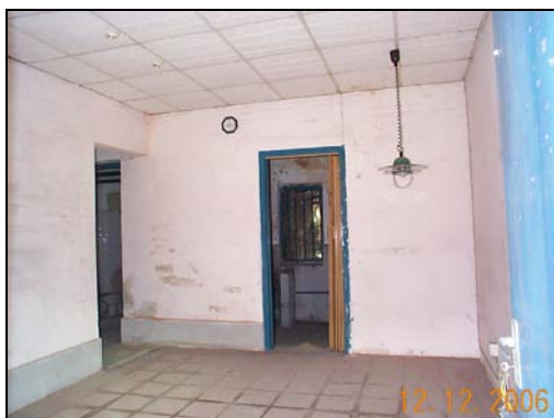
Suspended false ceiling at the east end room
