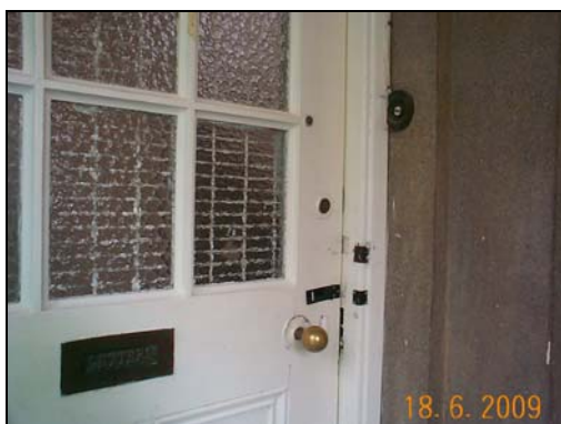
Ground floor quarter entrance door, the ironmongeries are brass letter box fascia plate, brass knob cylindrical door lock, cylindrical rim of the rim night latch, lock plate for the pad lock and peep eye
