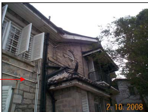
Water pipes fixed on the facade
