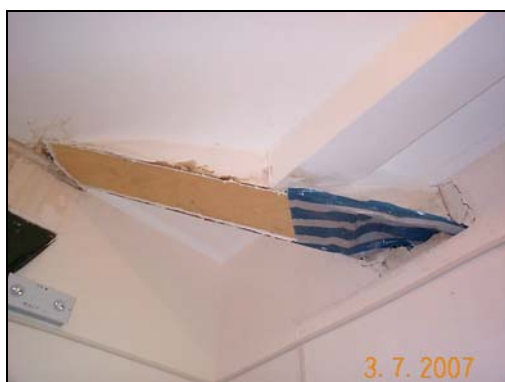
Roof water leakage at the ceiling of the corridor at first floor
