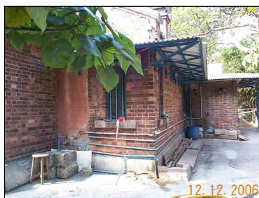
Later added canopy at rear elevation, east side
