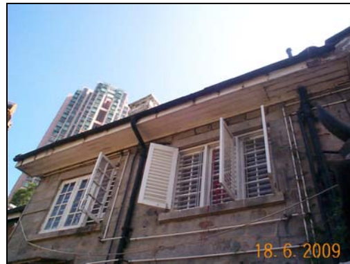
External view of windows on first floor – window on the right side open inwards and the left one open outwards
