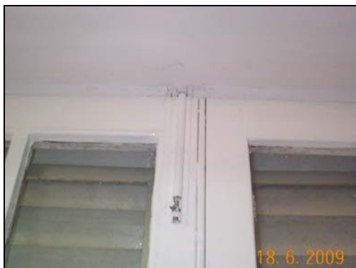
Vertical top bolt to French window at first floor balcony
