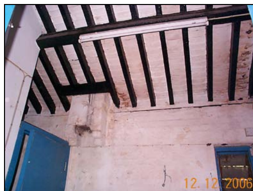
Timber purlin supporting the battens at the rear service room
