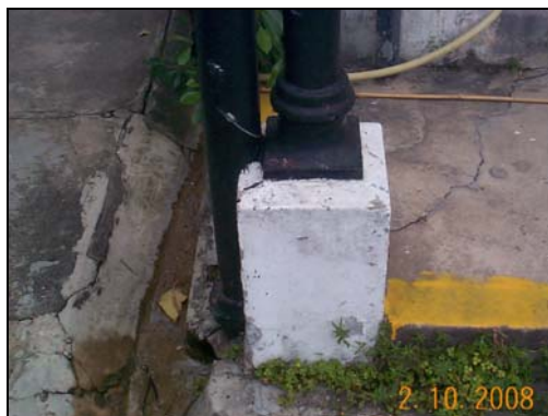
The shoe of the cast iron downpipe
