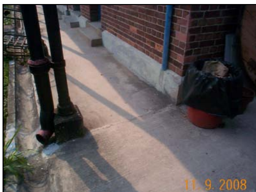
Cast iron pillar (lower part) and rainwater downpipe
