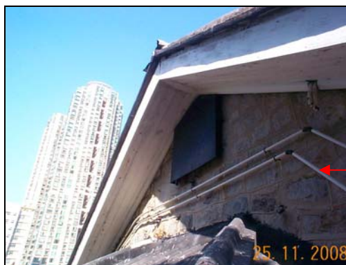
Water pipes fixed on the facade
