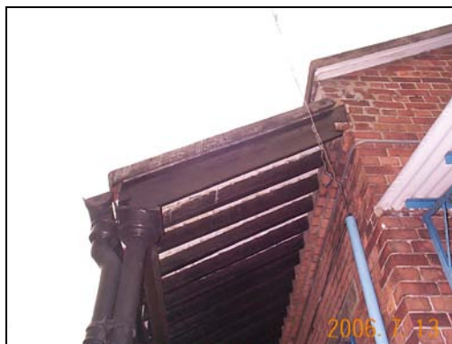
The timbers battens are supported by the timber purlin on the open side and the red facing brickwork cornice on the wall side
