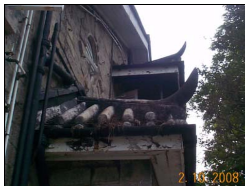
The “ox horn” at the end of the hip ridge at the roof to the entrance porch and the first floor balcony
