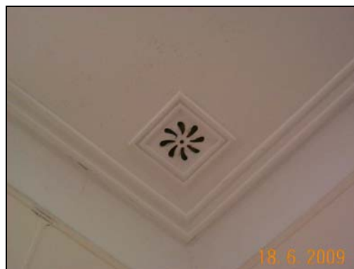
The cove ceiling border, cornice and grille pattern at the corner
