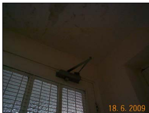
Ground floor quarter entrance door – the surface mount door closer
