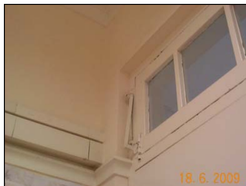
The lever arm catch of the top hung fanlight
