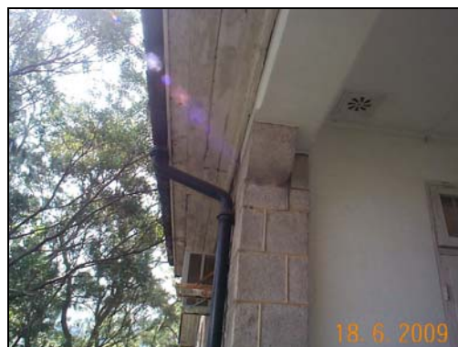
The pattern grille at one of the corners at ceiling of first floor verandah
