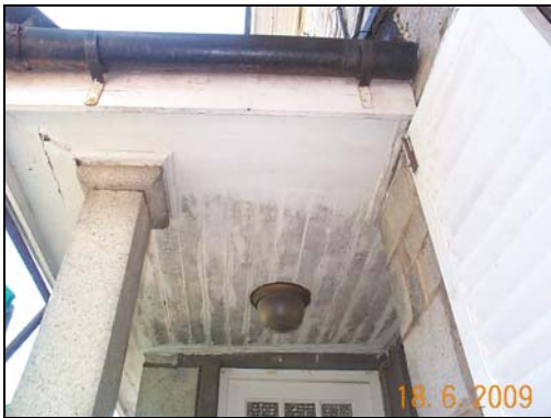
The timber false ceiling at ground floor entrance porch
