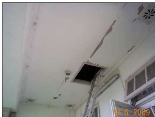
The timber false ceiling at first floor verandah
