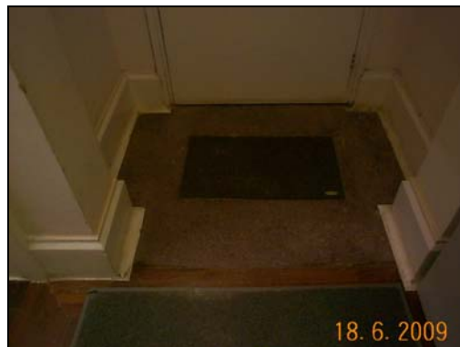
The floor mat well at the rear side of the ground floor quarter entrance
