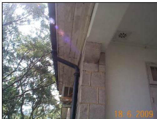
The soffit panel of the projecting roof eaves and fascia board at rear elevation
