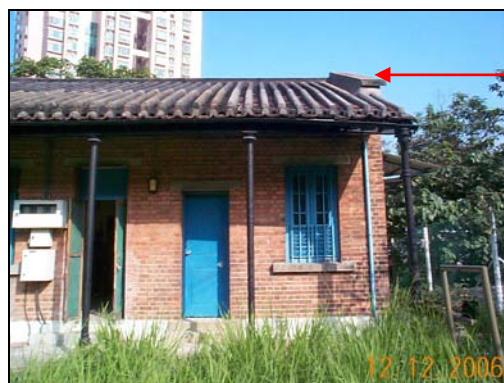
Granite coping on top of east gable wall
