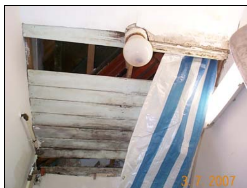
Roof water leakage at the ceiling of the toilet at first floor
