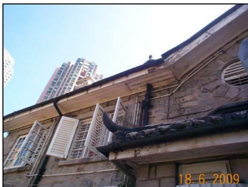
The soffit panel of the projecting roof eaves and fascia board at facade
