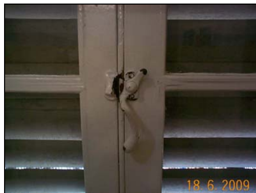
Lever handle lock to French window at first floor façade balcony
