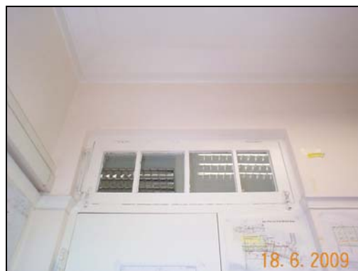
The top hung fanlight of an internal door
