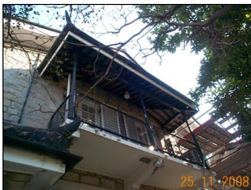
The “ox horn” at the end of the hip ridge at the roof to the entrance porch and the first floor balcony
