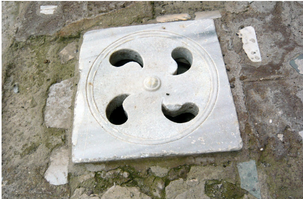
The uncovered floor drain made of marble is preserved in-situ and exposed for viewing. (Source: Yu Ka Sing 2012)
