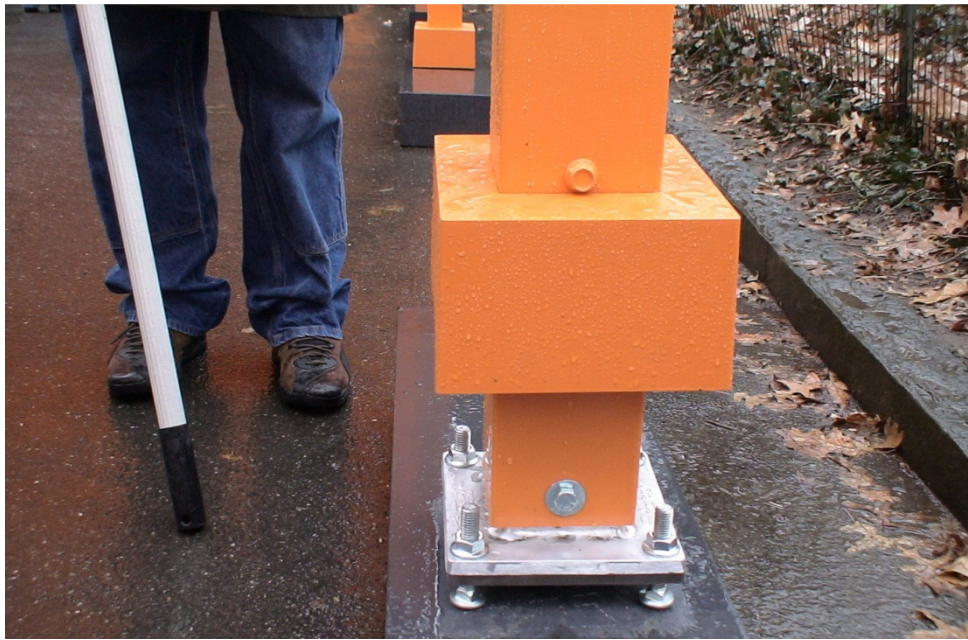
The cover of the footing is lifted up to reveal a design that does not involve invasive action at the pavement level. (Source: Yu Ka Foon 2005)
