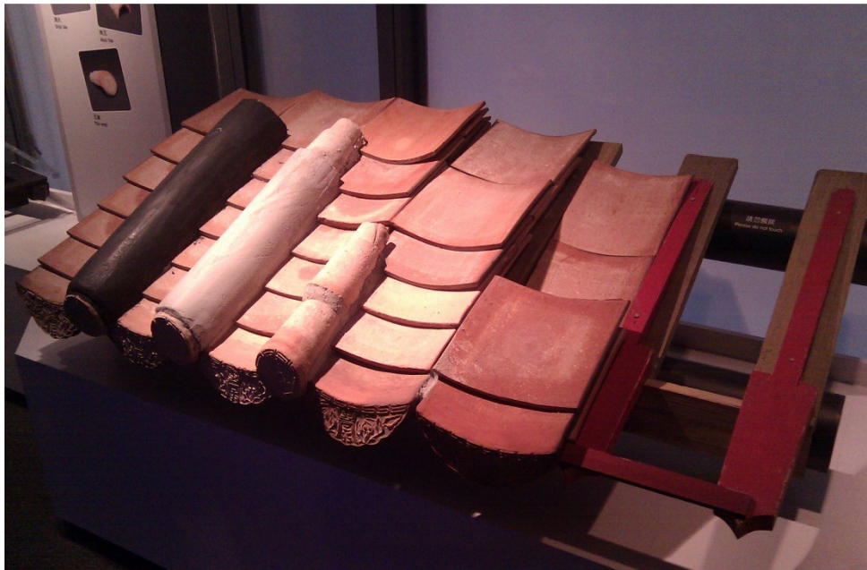
A full-scale model of traditional Chinese tiled roof at Heritage Discovery Centre demonstrate the composition and construction . (Source: Yu Ka Sing 2013)
