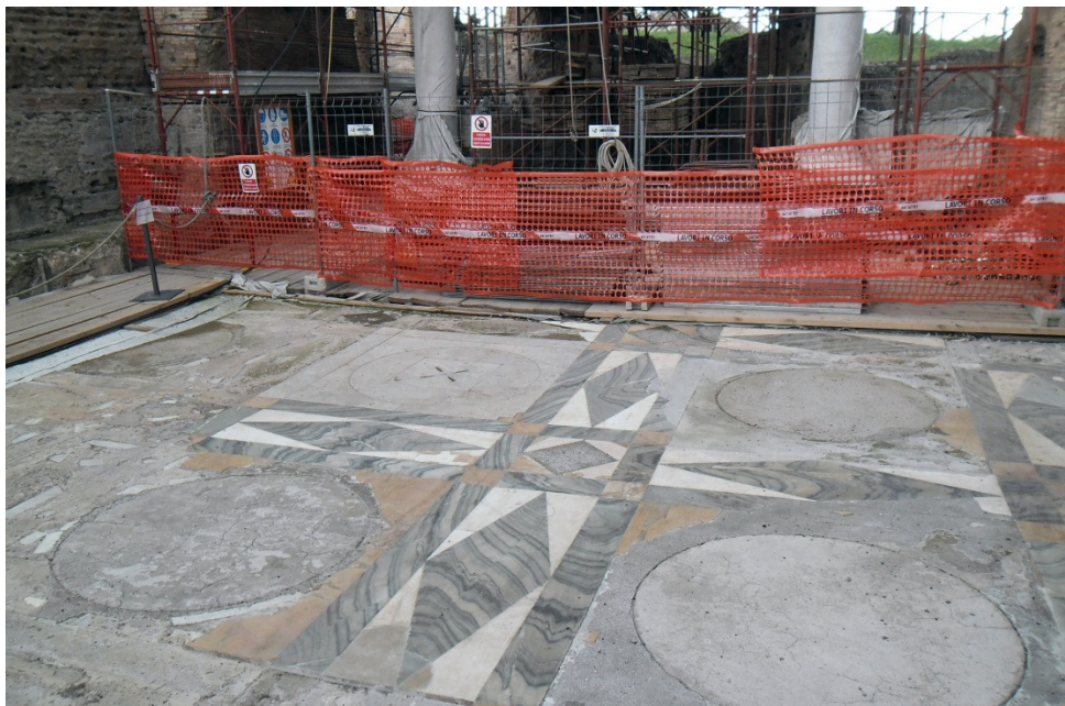
The magnificent marble floor that is entirely exposed is repaired to prevent further deterioration. Access by public is prohibited. The ruins are well protected during structural reinforcement works. (Source: Yu Ka Sing 2012)
