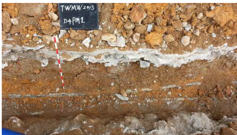
Photo B9 Northwest Section of D4PM2. Existing cables at the bottom of the trench and the water main is laid on top of the cables.
