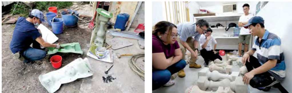
Fig. 15 The project team inspects and supervises the fabrication of newly-cast cement balusters to ensure they match the originals in terms of appearance, materials, colour, texture and craftsmanship.
