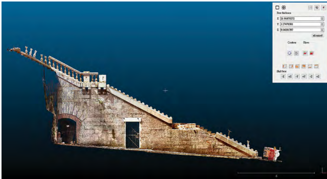
Fig. 11 A point cloud of the steps after the damage to them.
