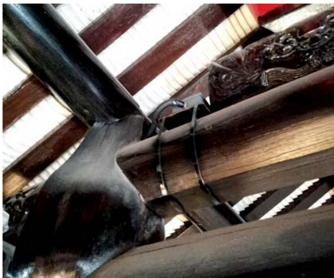
Figure 8 Vibration Monitoring Point and Distribution
