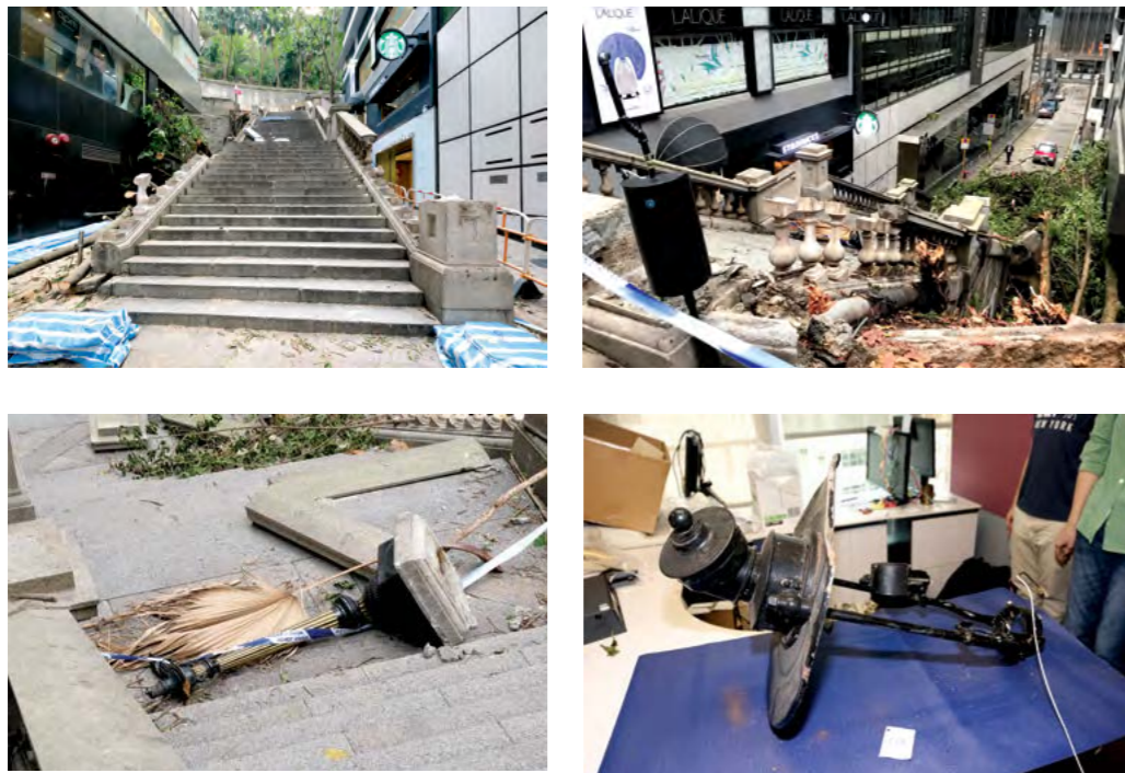
Fig. 6 The Monument was seriously damaged by the collapse of a large tree. The gas lanterns were deformed, and the cast iron column was broken into pieces.
