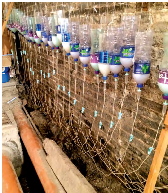
Figure 8 Damp-proof-course injection through gravity dripping Photo taken by the author
