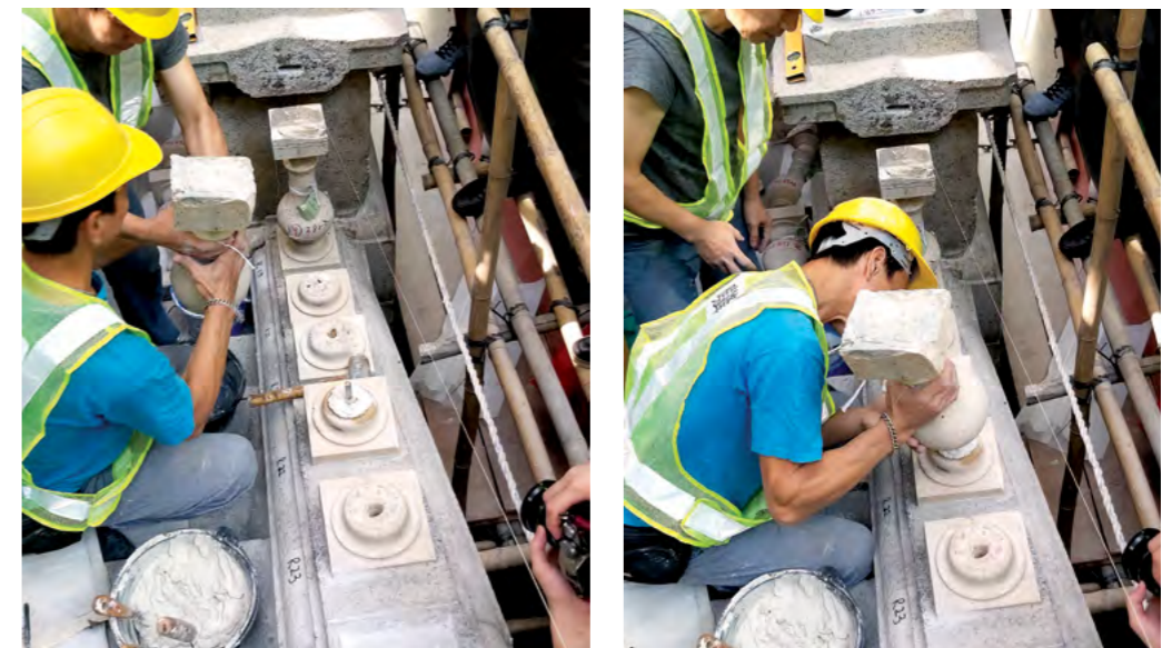
Fig. 17 Stainless steel rods are inserted into the balusters to strengthen them.
