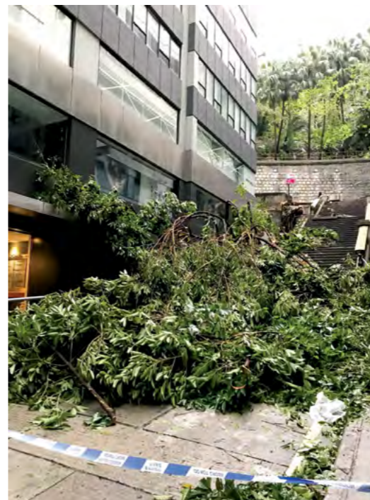
Fig. 1 The Duddell Street Steps and Gas Lamps were seriously damaged when Super Typhoon Mangkhut hit Hong Kong in September 2018.
