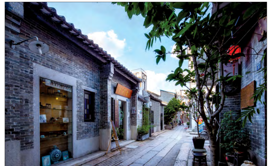
Figure 14 An ordinary lane after renovation
