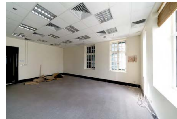
Figure 15 New accessible lift. Top: Condition before this project: A room at the northern corner of the building, which was used as an office in the Court of Final Appeal era. Bottom: After intervention: The design idea of transparency is to allow natural daylight through the surrounding windows to the lift car. [Source: Design 2 (HK) Limited]
