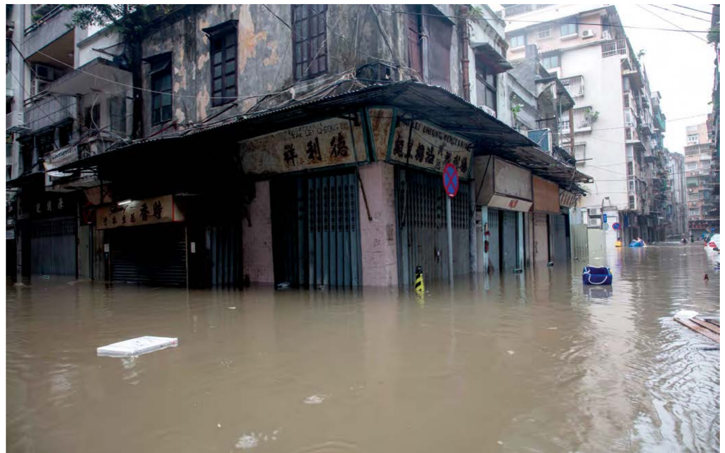
Figure 4 Flooding and seawater intrusion impacted in Macao during Typhoon Hato Source: Photo taken by Chan Hin lo
