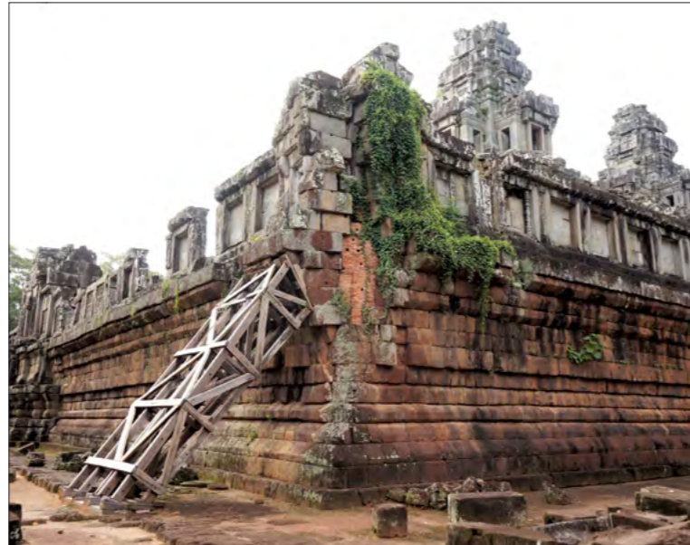
Fig. 3 Northwest corner and corner tower of the second floor of the Ta Keo Temple before restoration Source: China Academy of Cultural Heritage
