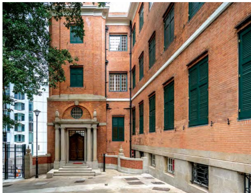
Figure 12 Restoration of entrance portico.
