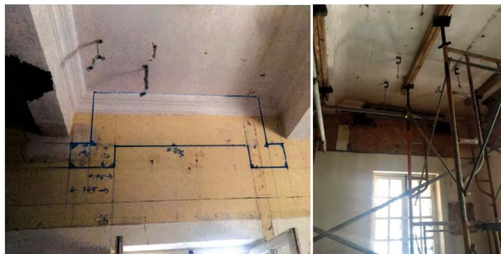
Figure 14 Fixing new steel structural members to original load-bearing brick walls.
