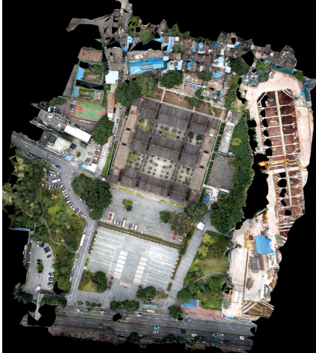
Figure 2 Bird's Eye View of the Current Situation around the Chen Clan Ancestral Hall
