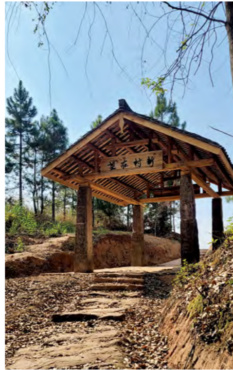
Figure 16 The pavilion after restoration.
