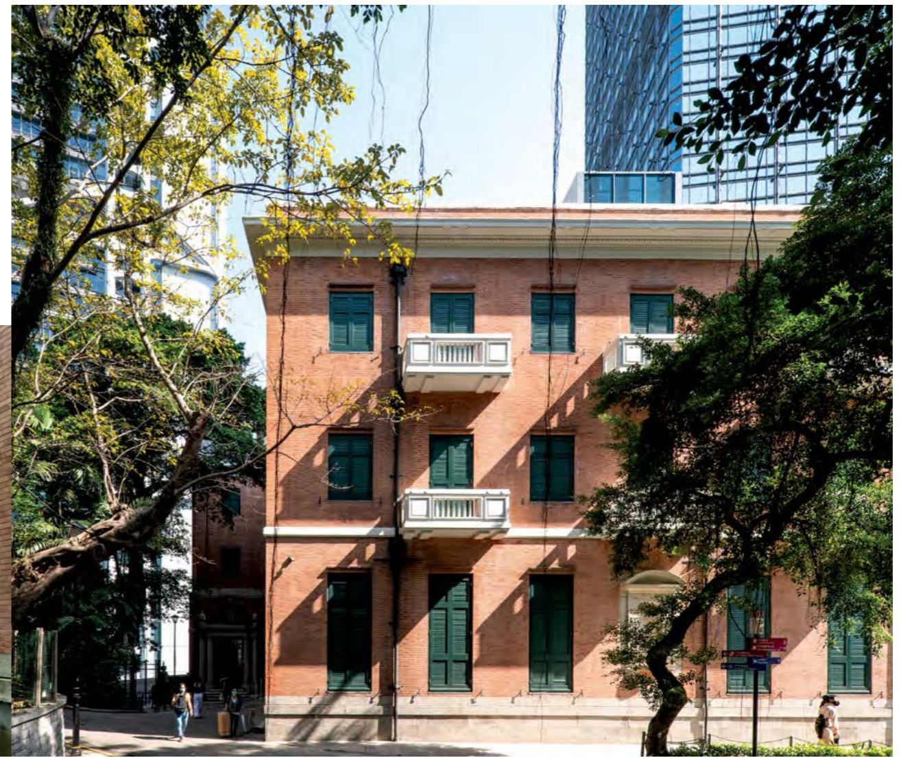
Figure 13 Southwestern façade – reconstructed timber shutters in green. [Source: Design 2 (HK) Limited]
