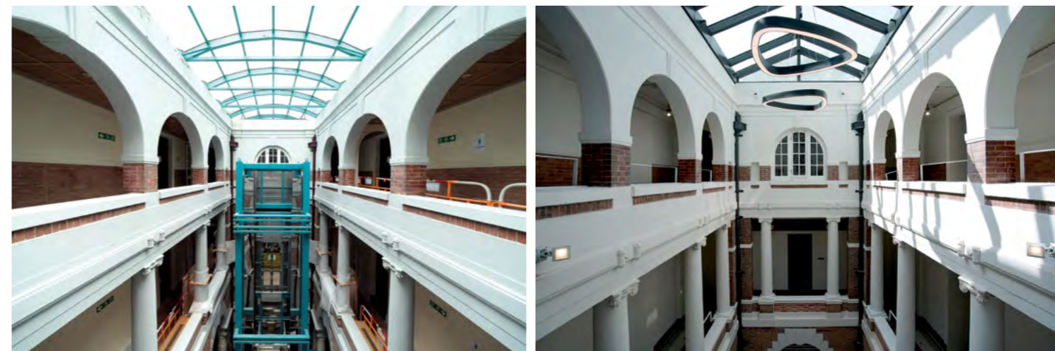
Figure 10 Restoration of internal courtyard. Left: Condition before this project: A lift shaft made of steel was added to serve the G/F and 1/F only when the building was converted to the Court of Final Appeal. Right: After restoration: The old skylight is replaced by a pitched one and the old lift shaft was removed. [Source: Design 2 (HK) Limited]
