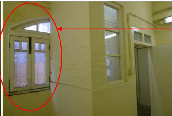
Existing windows beside ST-2 can be protected by adding fire rated board at the rear.
