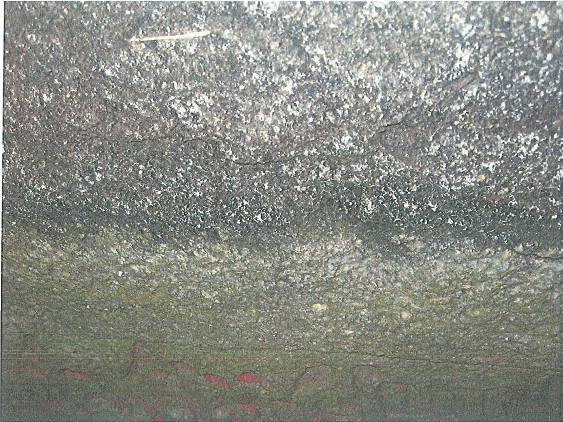
Photo 1: Interface between cleaned and uncleaned surface
