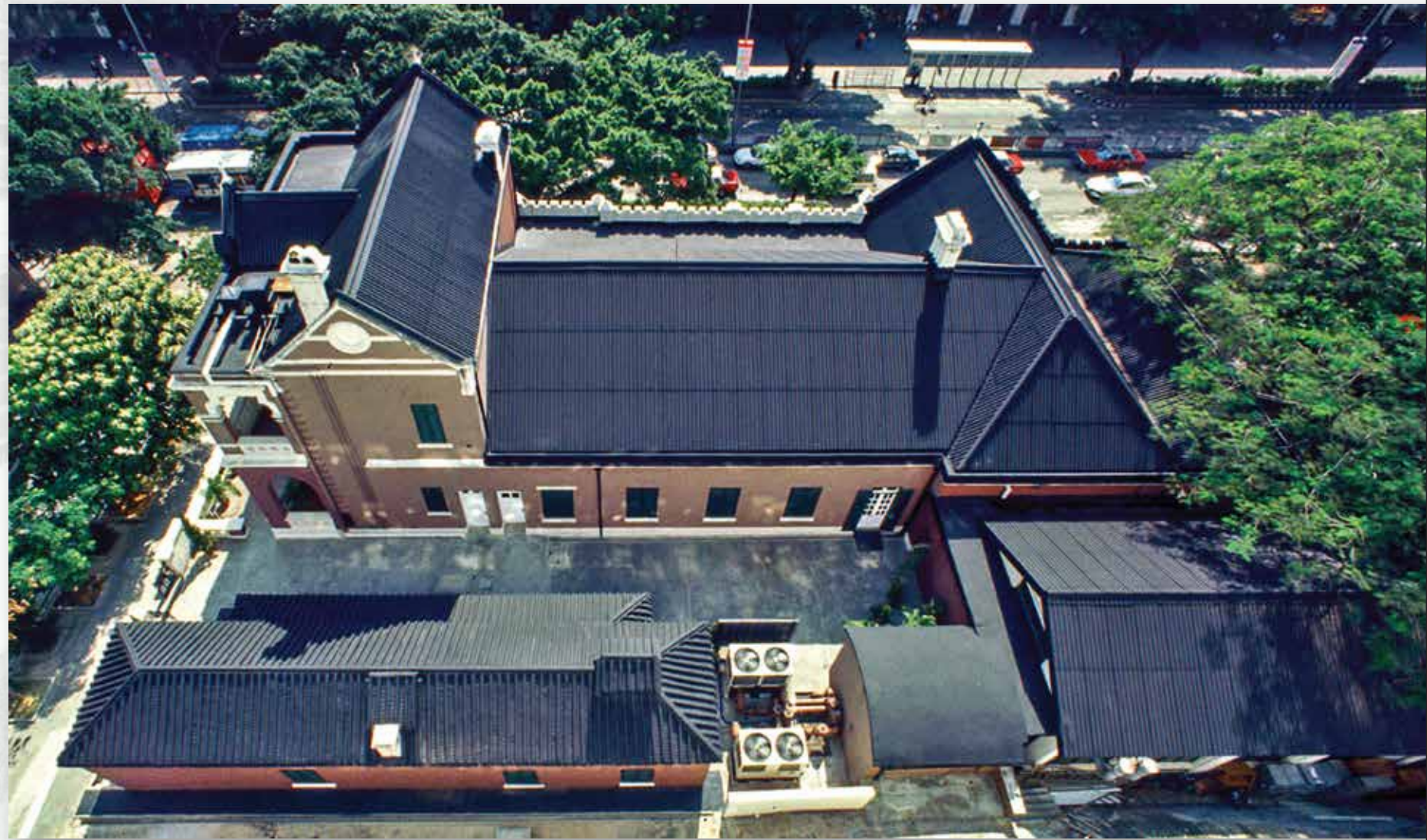
從高空俯瞰整個建築物，可見金字瓦頂及煙肉。 Overview of the building showing its pitched roofs and chimney stacks.
