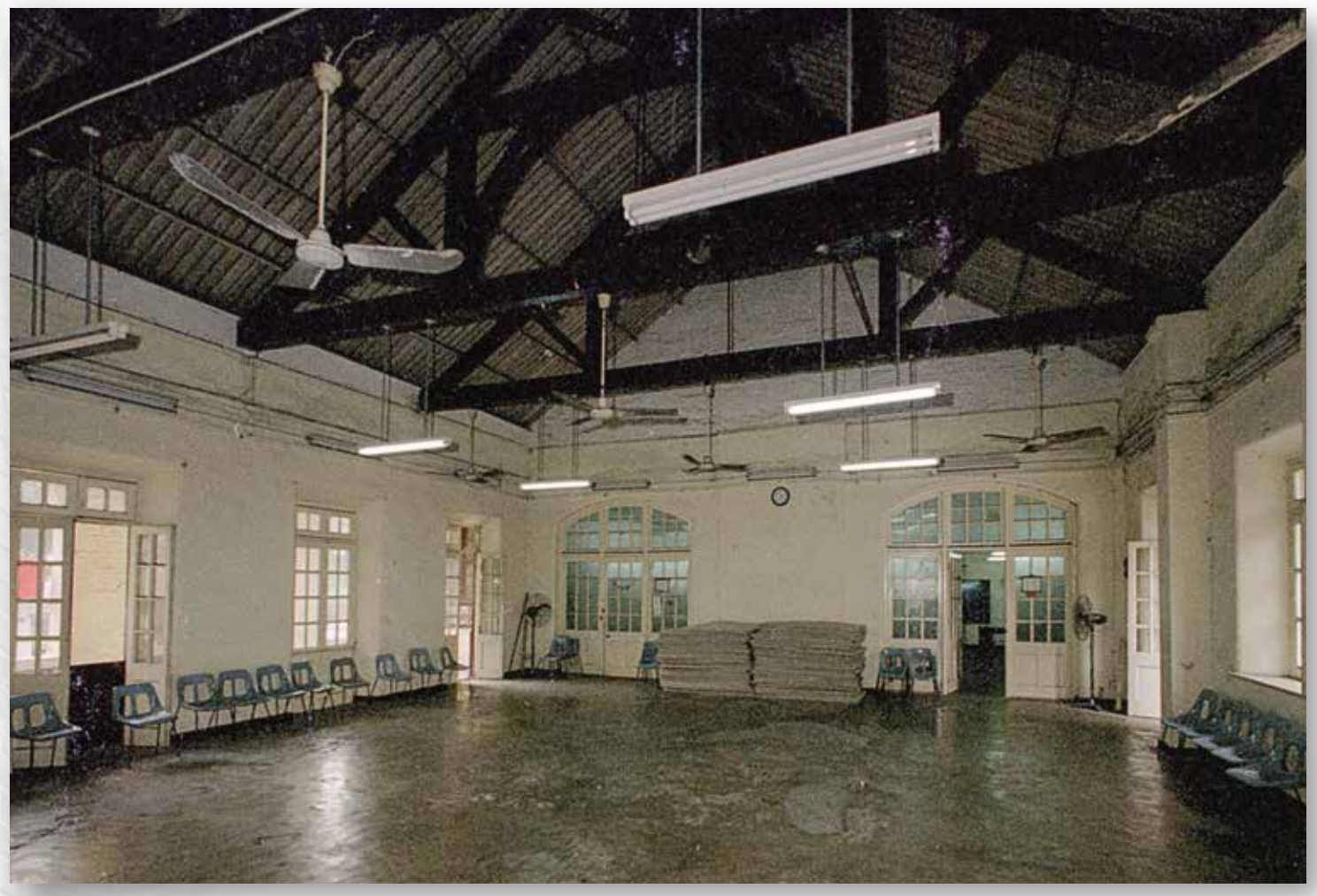
昔日的學校禮堂，樓底很高，有助通風及防潮。 The old school hall with its high ceiling to improve ventilation and damp-proofing.
