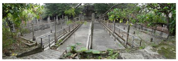
Proposed rain shlter, retained feeding trough and new RC feeding trough.
