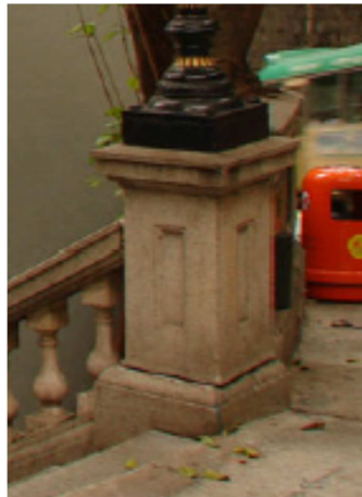
Fig.101: Stonework of the Duddell Street Steps
