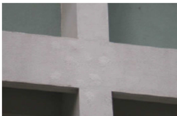
Fig.29: Concrete repairs on the West Wing
