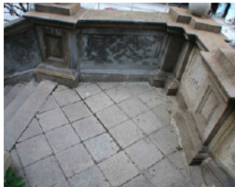
Fig.35: Concrete repairs and gaps in the paving of the Battery Path steps adjacent to the French Mission Building
