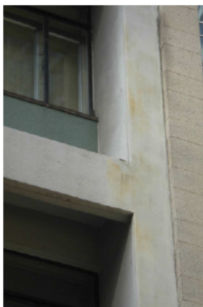
Fig.31: Staining on the West Wing
