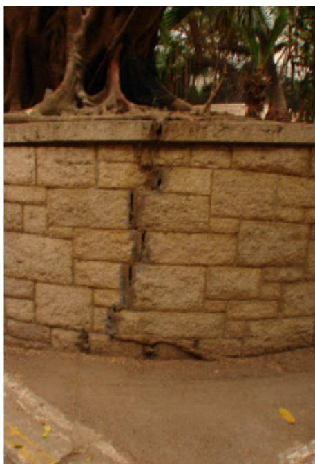
Fig.32: A large crack in a retaining wall of a shrub bed
