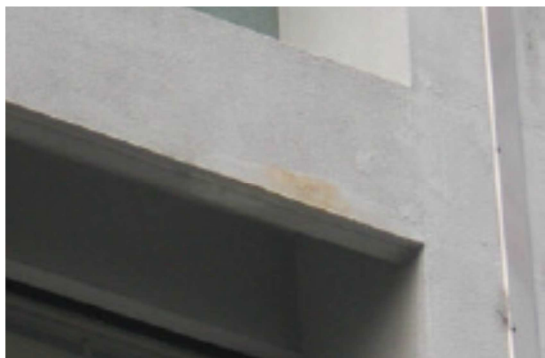
Fig.30: Staining on the West Wing
