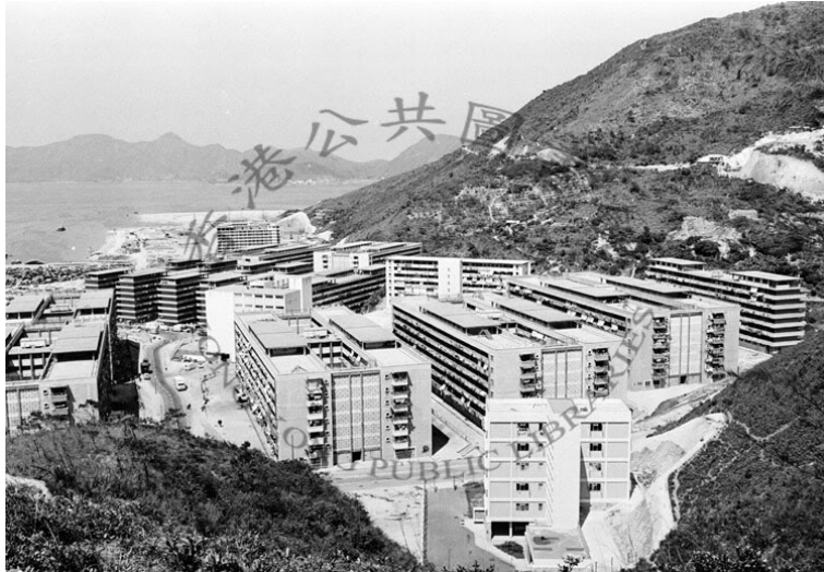
Fig. 27. The blocks of Resettlement District in Chai Wan, H-Shaped Mark I blocks can be seen at the back, and Mark II blocks with inner courtyards are closer to the bottom of the picture, 1964.
