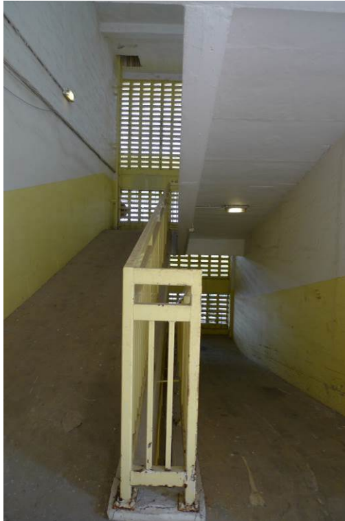
Fig. 73. The ramp that provides vertical access for bulky items.
