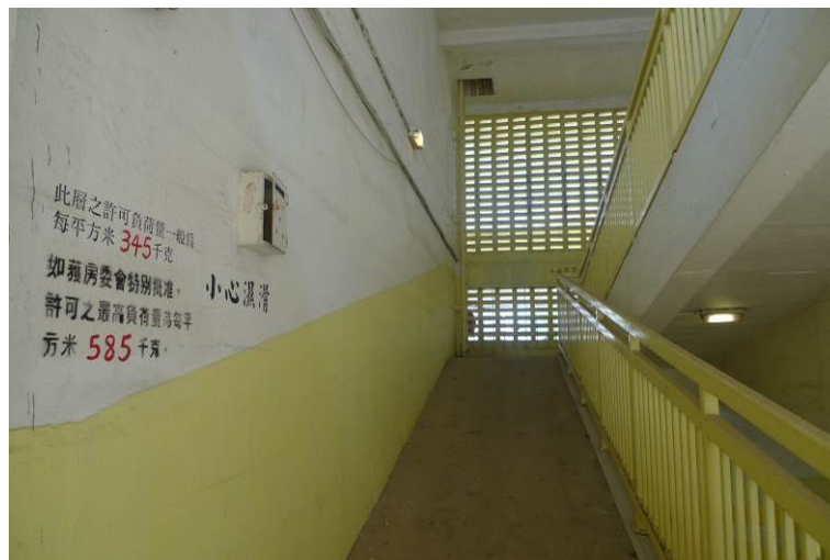
Fig. 99. Access ramp with window openings to provide ventilation.
