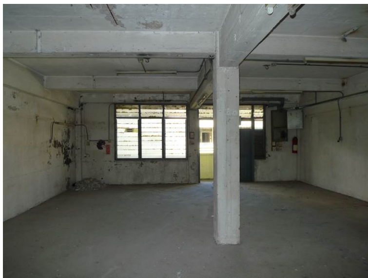
Fig. 69 Column, beam and slab construction.
