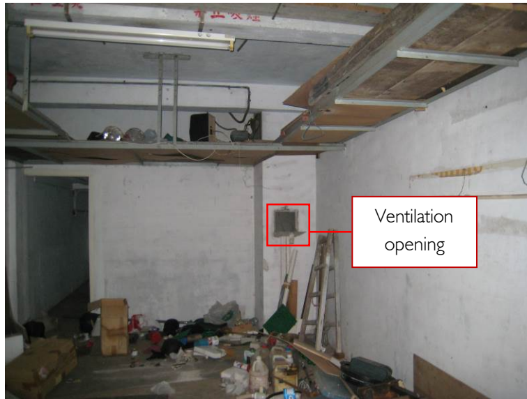
Fig. 83. Ventilation opening at a flat on the third floor.
