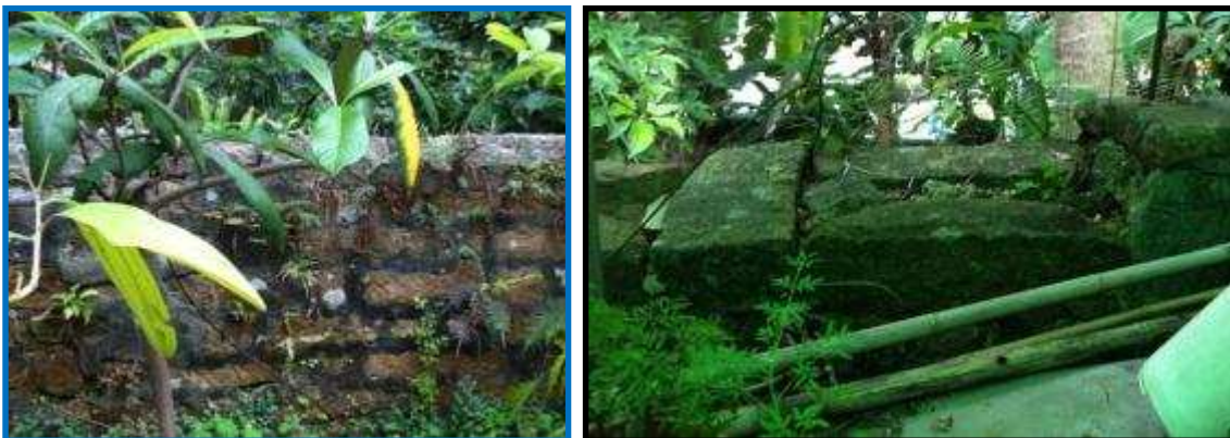
Figure 18: Photo of existing stone wall within the Site of FWPS and a close-up of the damaged capping stone Source: photo by the author
