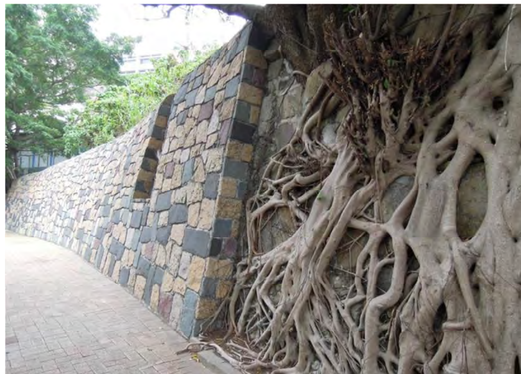
The retaining wall along the Pok Fu Lam Road leading from the Main Office Building to the Bethanie is believed to be the original boundary wall of the Mains of Old Dairy Farm, while it has been reinforced and covered up by a “new wall”. (Source: China Point)
