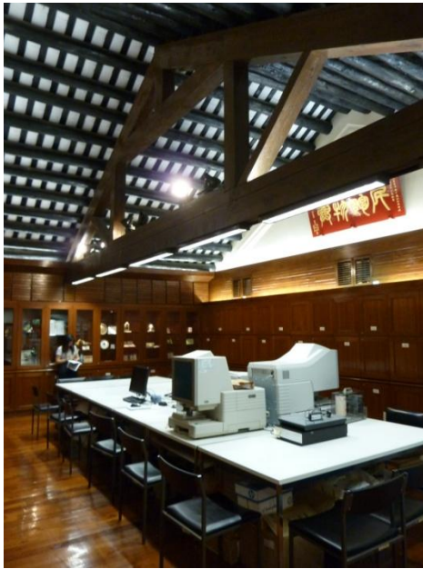
Western-style timber truss system supporting the pitched roof.
