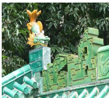
Ceramic ridge details with geometric ends and dragon-fish decors
