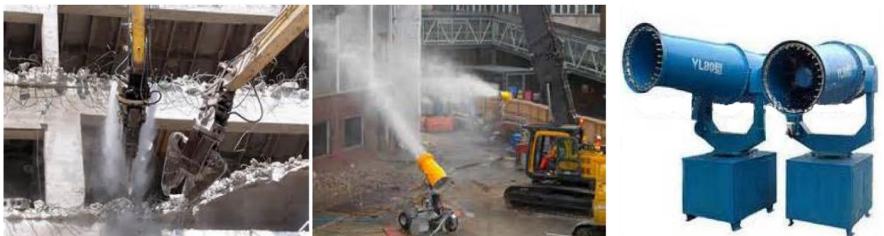
Fig. 13 – Additional protective measures against dust deposition – Atomized spray device
