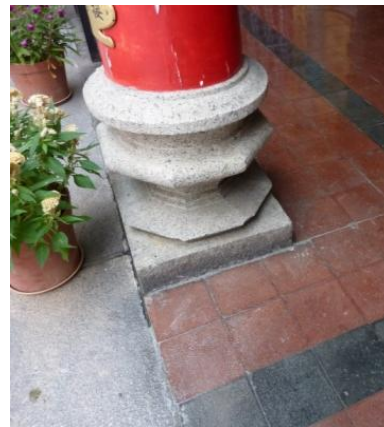
Granite column base with the cement tiles detail
