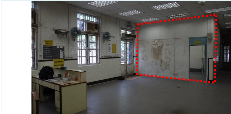
Fig 21. The existing photo of Lady Ho Tung Welfare Centre in 2016. The part of the later-added fiberboard partition wall is retained in-situ (highlighted in red). Edited by Hannah Liu
