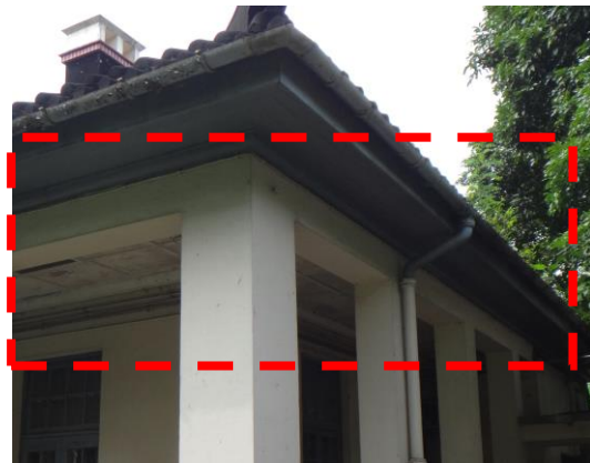
Fig 32. The horizontal concrete beam spanning between the concrete columns
