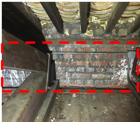
Fig 31. The timber trusses are sited on the brick wall above the horizontal concrete beams at south.
