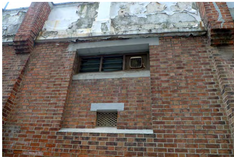
Fig. 116. Louvre windows and metal grating on the wall facing the 1 st plateau.
