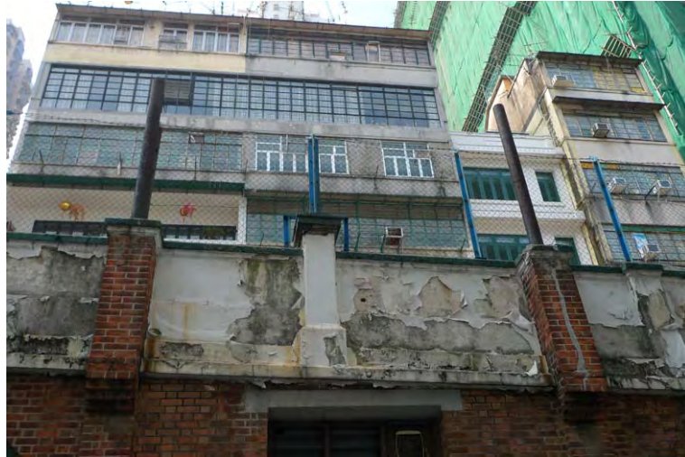
Fig. 115. Two wrought-iron pipe shafts for ventilation.
