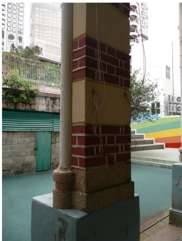
Internal face of banded column
