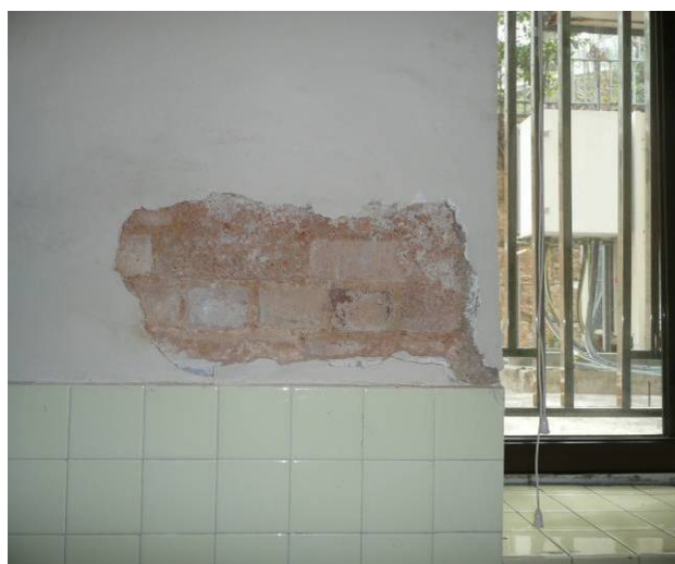
Evidence of original wall materials – Ground Floor
