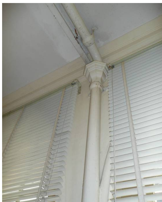
Internal drain pipe
