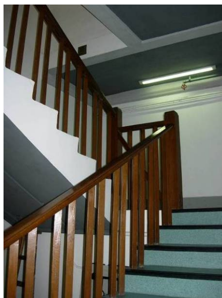
Timber balustrading to staircase in Eliot Hall HKU
