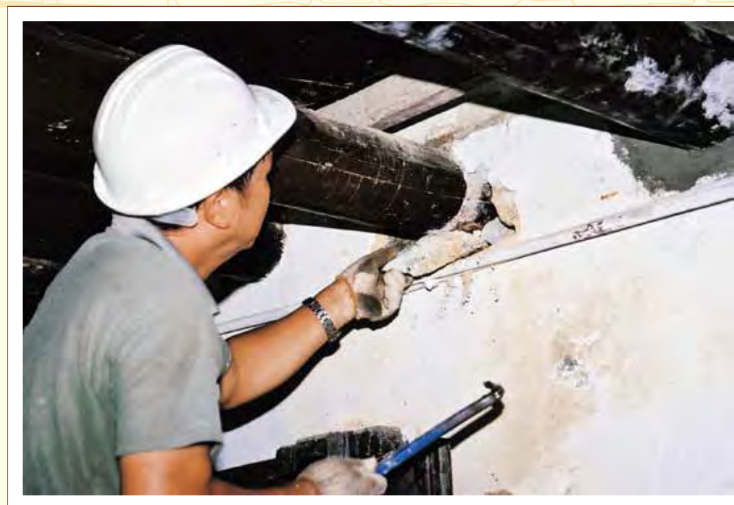
更換損毀的樑條 Replacement of defective purlin
