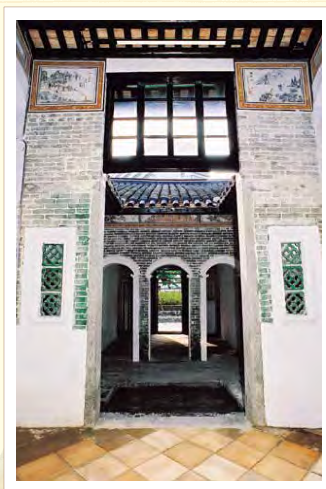
古屋地面以廣東大階磚鋪設成菱形圖案 The Old House is paved with Canton tiles in diamond patterns.
