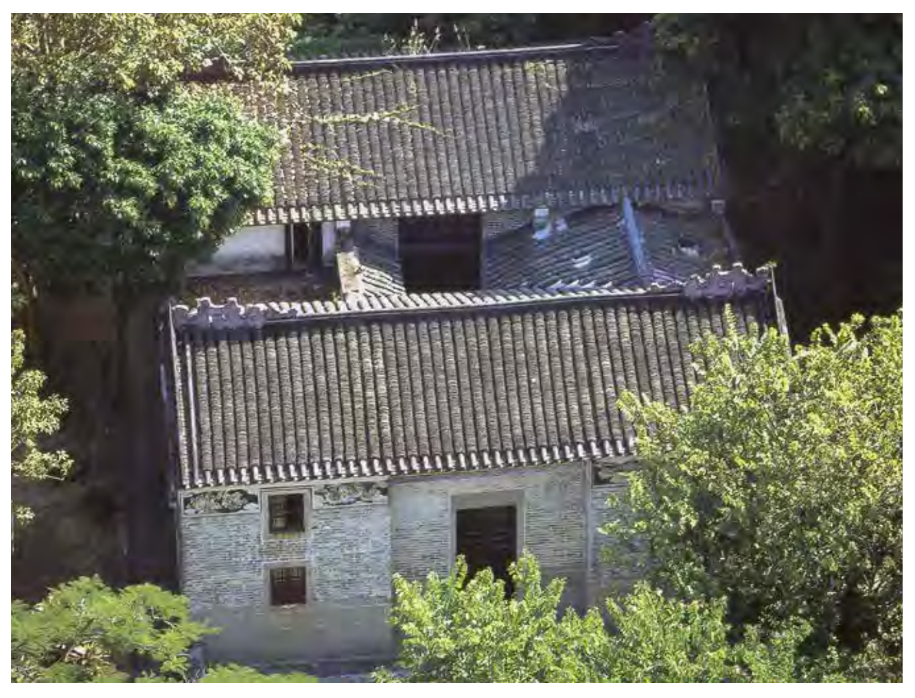
古屋為傳統客家的兩進一天井三開間式建築 Old House is a typical traditional Hakka residence having a layout of two-hall-one-courtyard with three bays.
