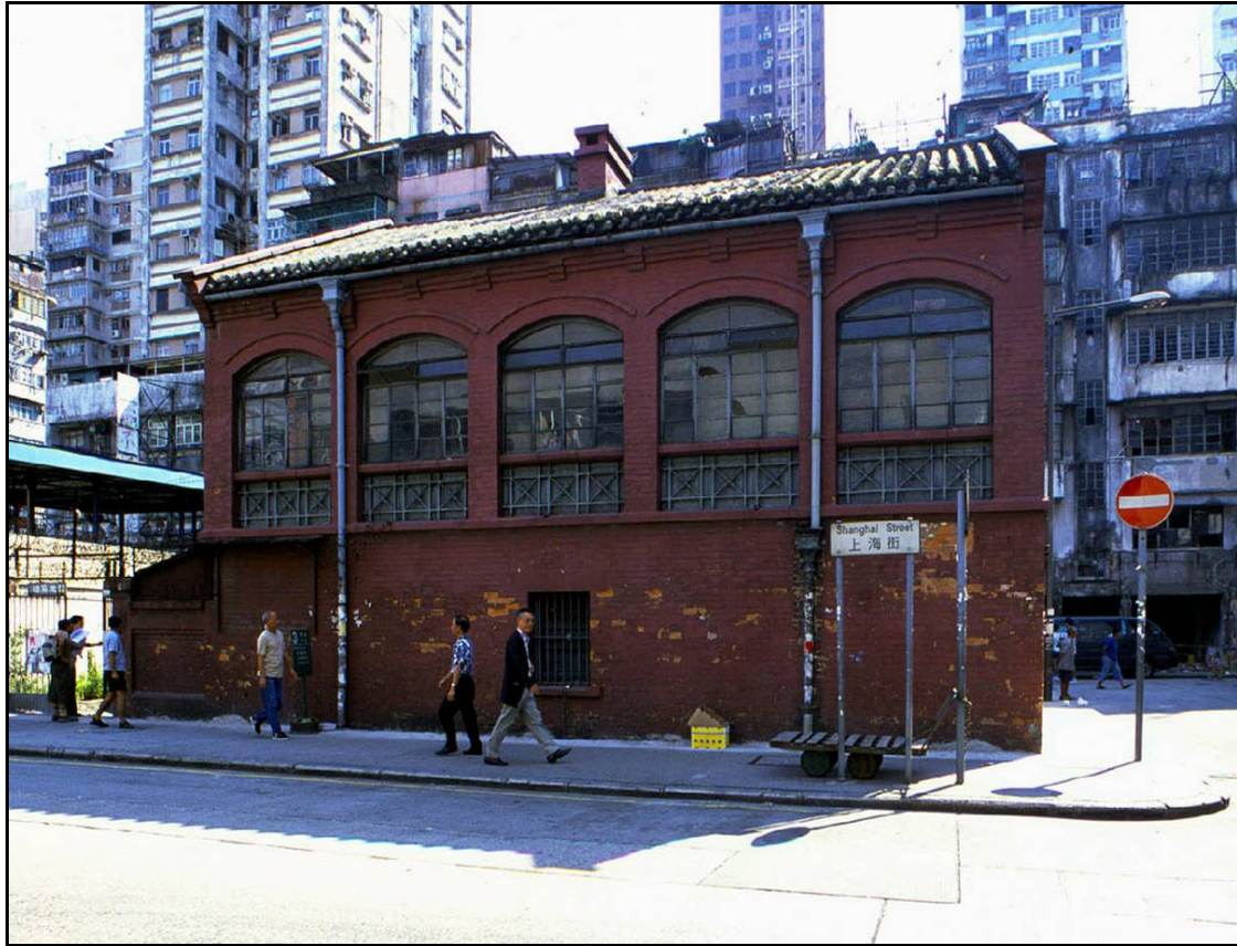
Fig. 8 The sole surviving building of the Yau Ma Tei Pumping Station complex as it appeared in 2000. (Source: Lee Ho Yin)
