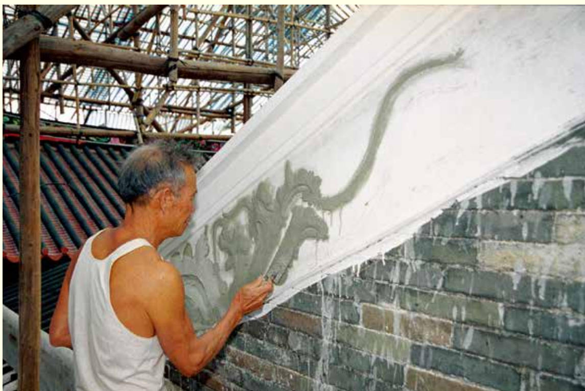
工匠於牆頭修復灰塑 Redecoration of plaster mouldings on wall frieze
