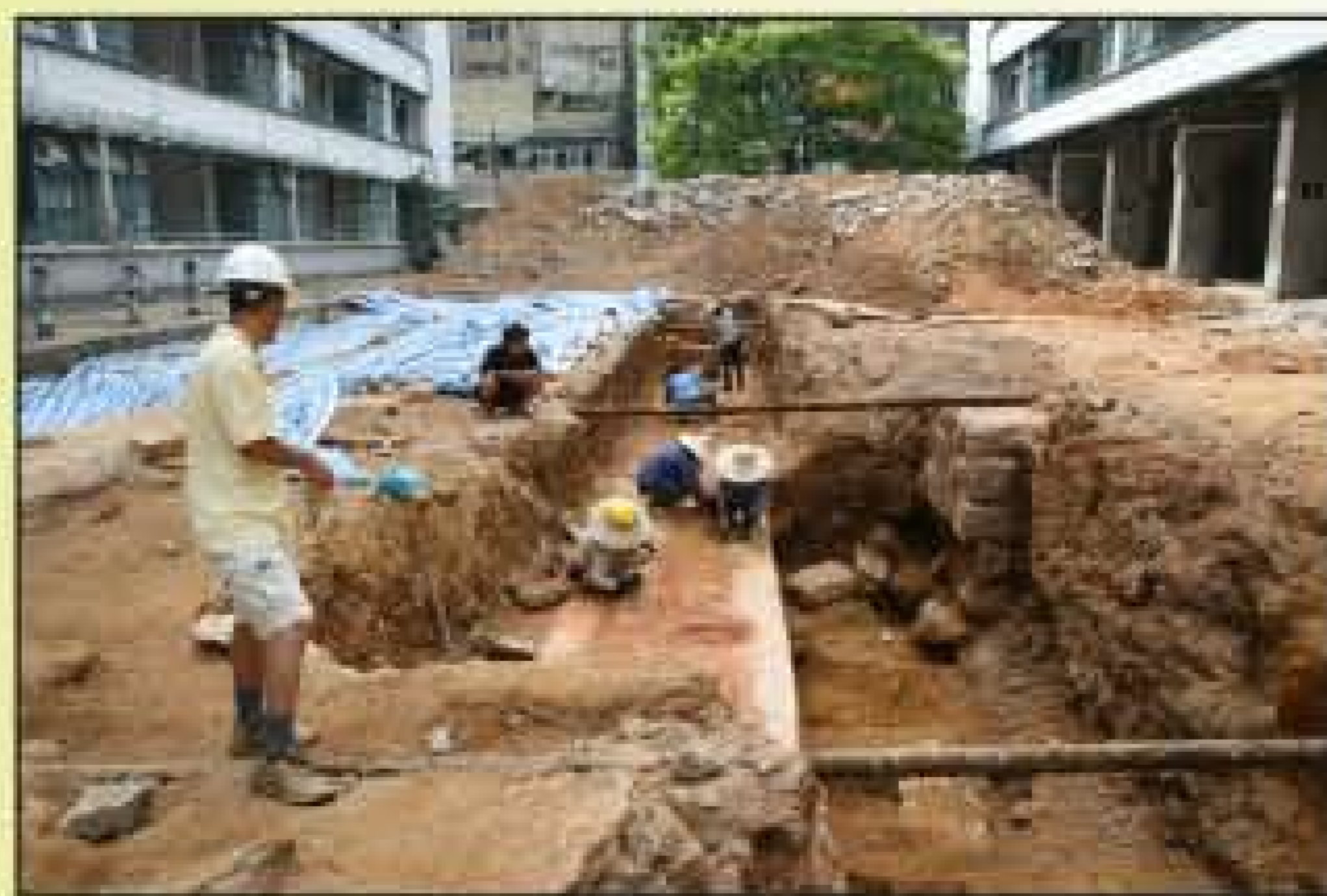
人手清理牆基9號 Stone Foundation No. 9 cleared by hand excavation
