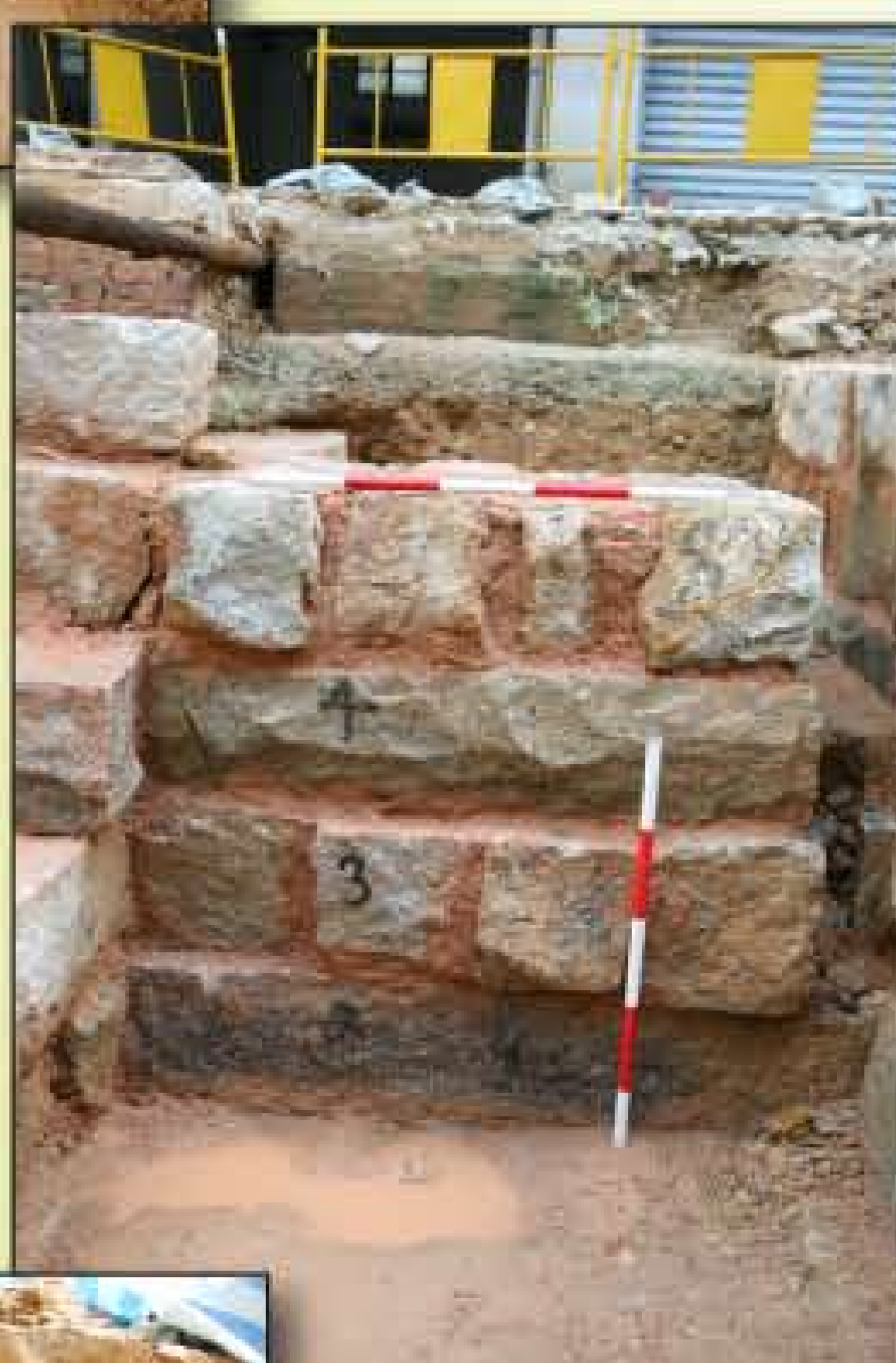
牆基3號南部的“2”、“3”、“4”及“5”墨跡 Inked marks “2”, “3”, “4” and “5” on the southern part of Foundation No. 3
