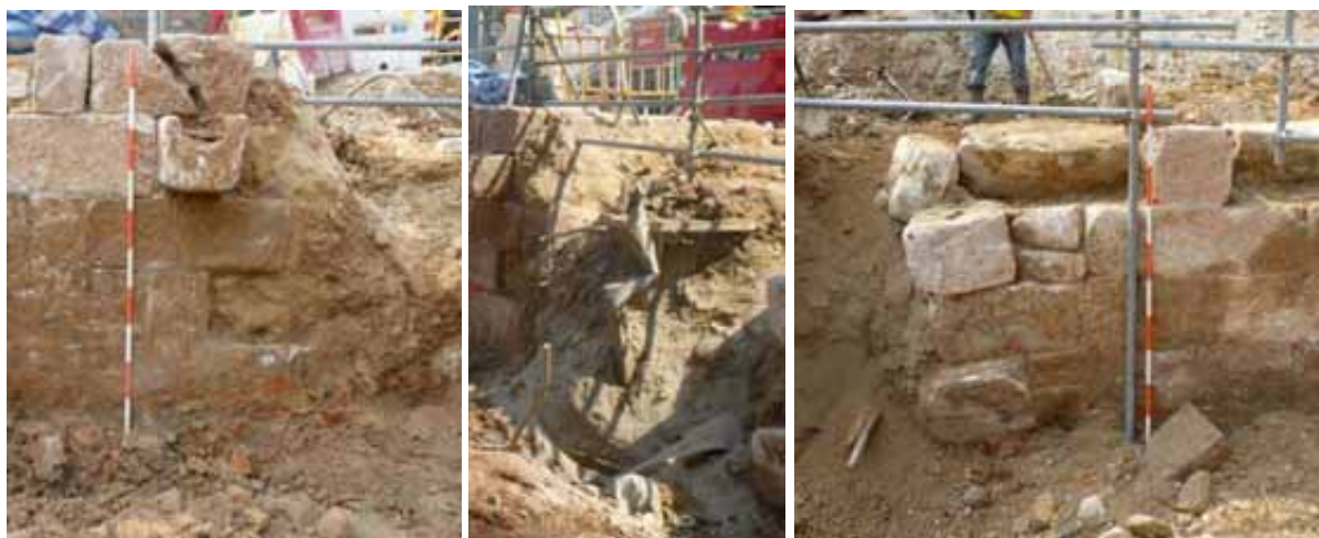
PLATE 13 a Plunge column sunk from surface level prior to excavations has dissected the seawall fragment and affected the condition of seawall; left and right shows seawall fragment on either side of the plunge column (centre photo)
