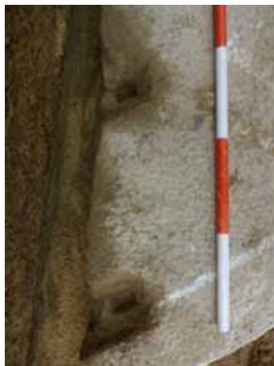
PLATE 5 Landing stone at the bottom of the seawall fragment; 'Lewis holes' detail on right
