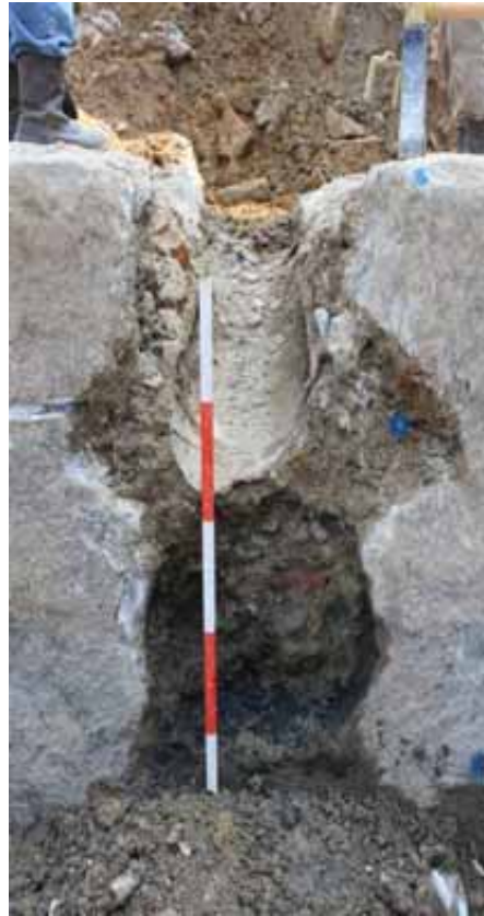
b. Circular stone sewage out let with later addition on top
