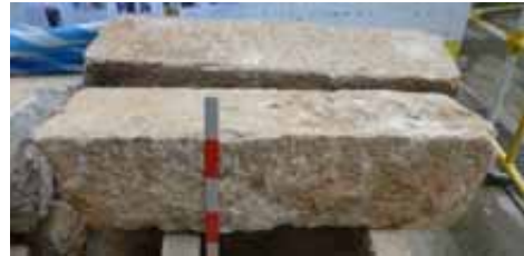
View of side of dressed stretcher block
