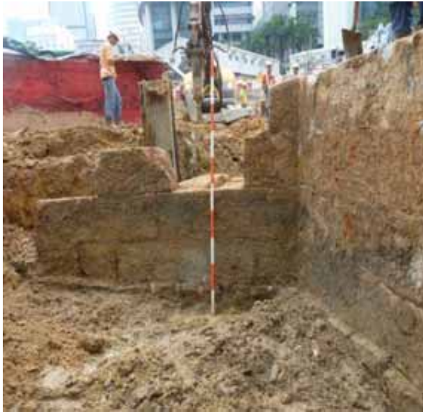
a. Seawall fragment curving to the north in the east; notice the inner structure of the seawall fragment
