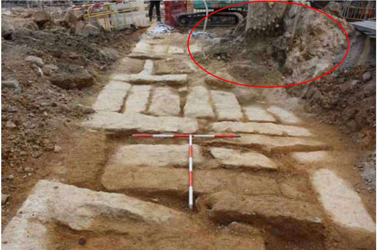
PLATE 13 b Plunge column sunk from surface level prior to excavations damaged the rear of the seawall fragment
