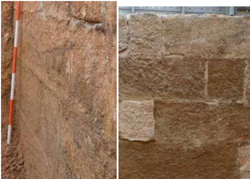
PLATE 3 Dressed granite blocks of the north façade of the seawall fragment
