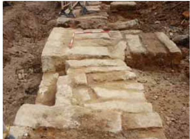
PLATE 2.f Uncovering 'row 4' with rear abutment
