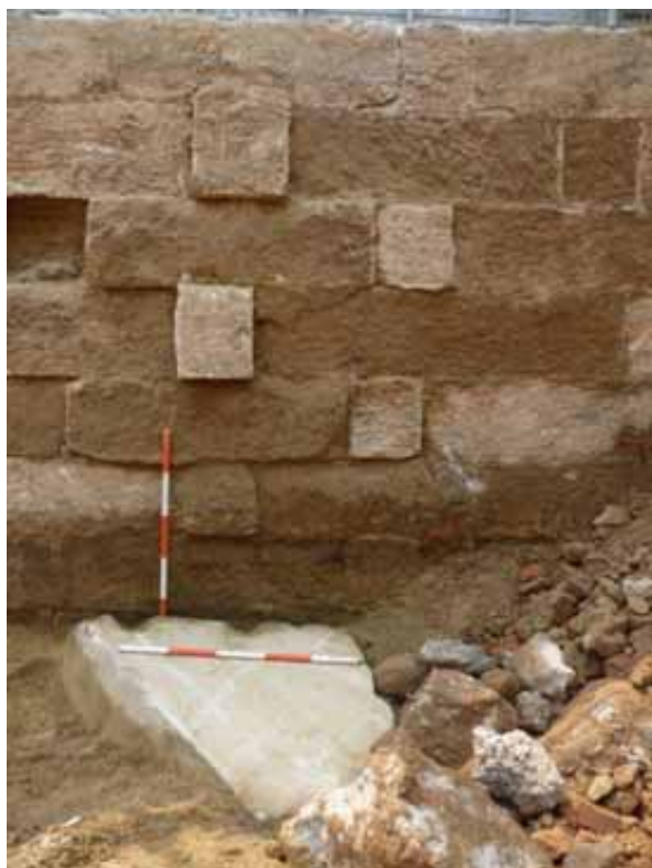
PLATE 5 Landing stone at the bottom of the seawall fragment; 'Lewis holes' detail on right
