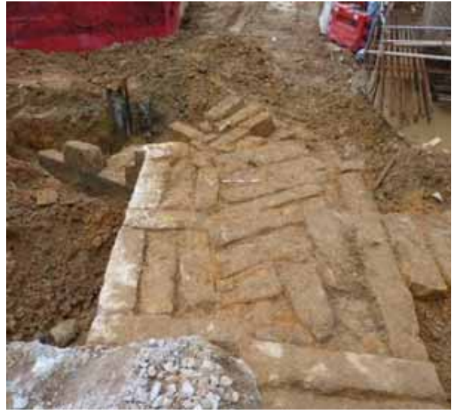
a. Seawall fragment curving to the north in the east; notice the inner structure of the seawall fragment
