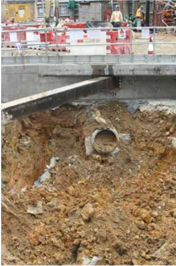
PLATE 19 Concrete casing and pipe from a previous development which cut the top of the well and leaves shaft and bottom on well
