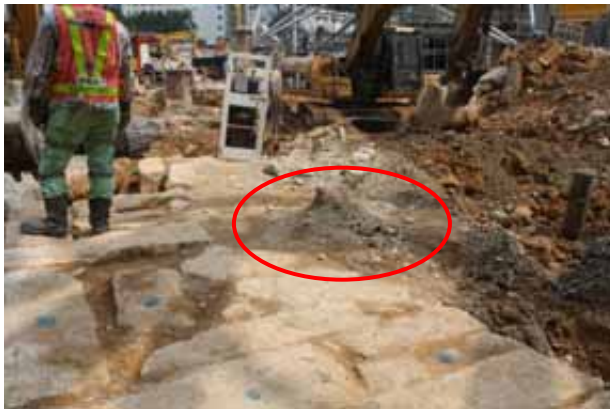
PLATE 13 c Thick rebar foundations part of previous MTRC Entrance/Exit 'E' construction damaged the rear of the seawall fragment
