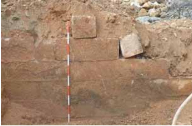
PLATE 3 Dressed granite blocks of the north façade of the seawall fragment
