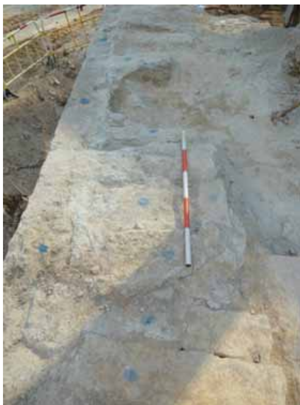
PLATE 11 Concrete on top of the seawall fragment in the eastern section
