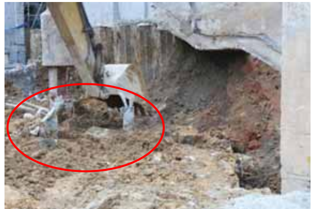
PLATE 13 c Thick rebar foundations part of previous MTRC Entrance/Exit 'E' construction damaged the rear of the seawall fragment
