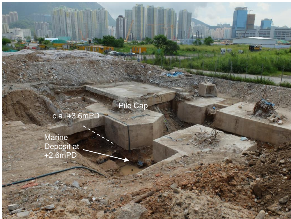
Figure 5.6 Pile Caps and Ground Beams at T14, T14a and T21.
