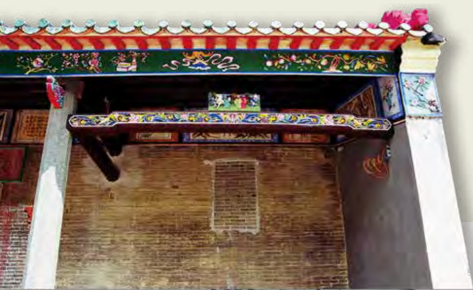
利用青磚封閉正面窗戶 Sealing the window on the facade with grey bricks
