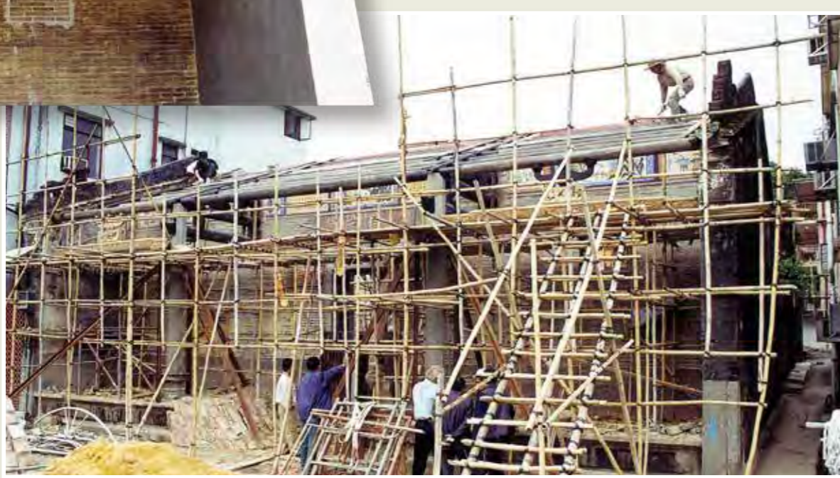
重鋪前進天面 Rebuilding the roof of the front hall
