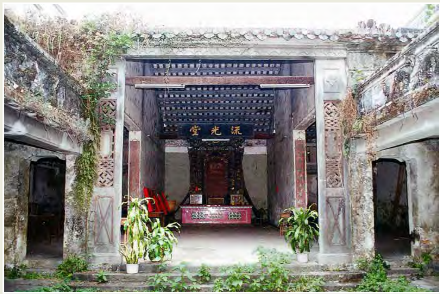
修復前敬羅家塾的內貌 Interior of King Law Ka Shuk before restoration
