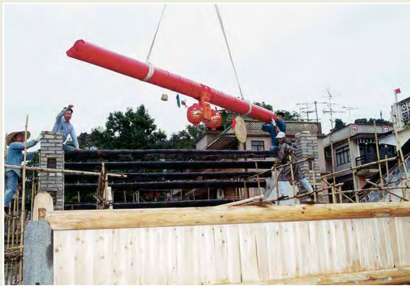
安裝主樑 Installation of the ridge purlin
