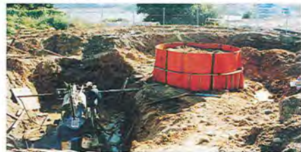
對唐窯遺跡進行加固和搬遷 To reinforce a Tang dynasty kiln structure before relocation.
