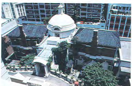
57. 香港大學孔慶慶樓外部 The Exterior of Hung Hing Ying Building, the University of Hong Kong
