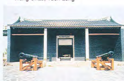
63. 前九龍寨城衙門，九龍寨城公園 Former Yamen Building of Kowloon Walled City, Kowloon Walled City Park
