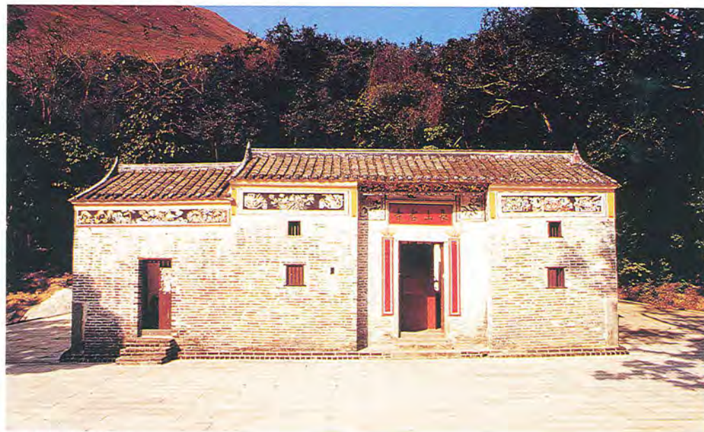
修復後的長山古寺 Cheung Shan Monastery after restoration.
