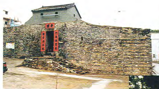
復修後的老圍 Lo Wai after restoration.
