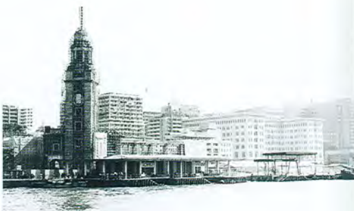
火車站於一九七八年拆卸 Demolition of Terminus in 1978.
