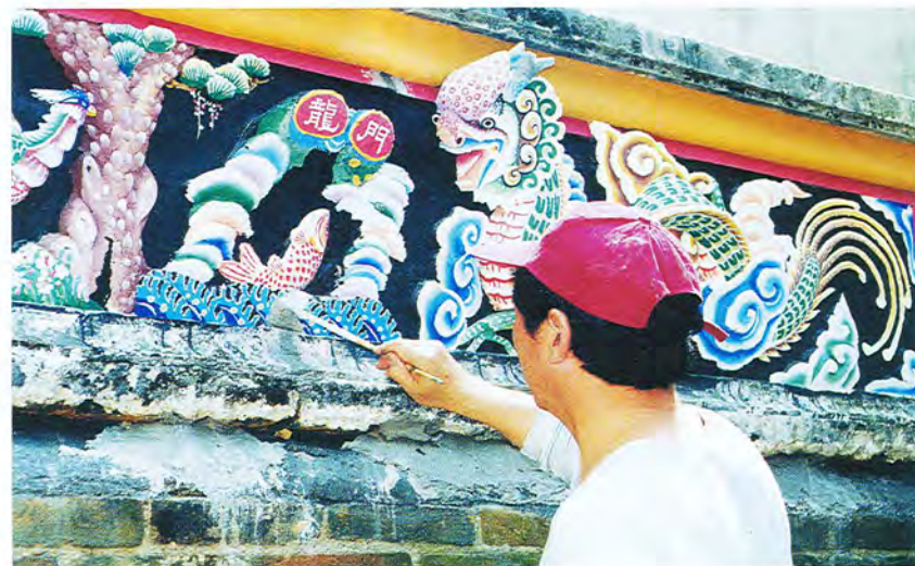
為敬羅家塾的泥塑重新上色 Repainting the moulded panel of King Law Ka Shuk Ancestral Hall.
