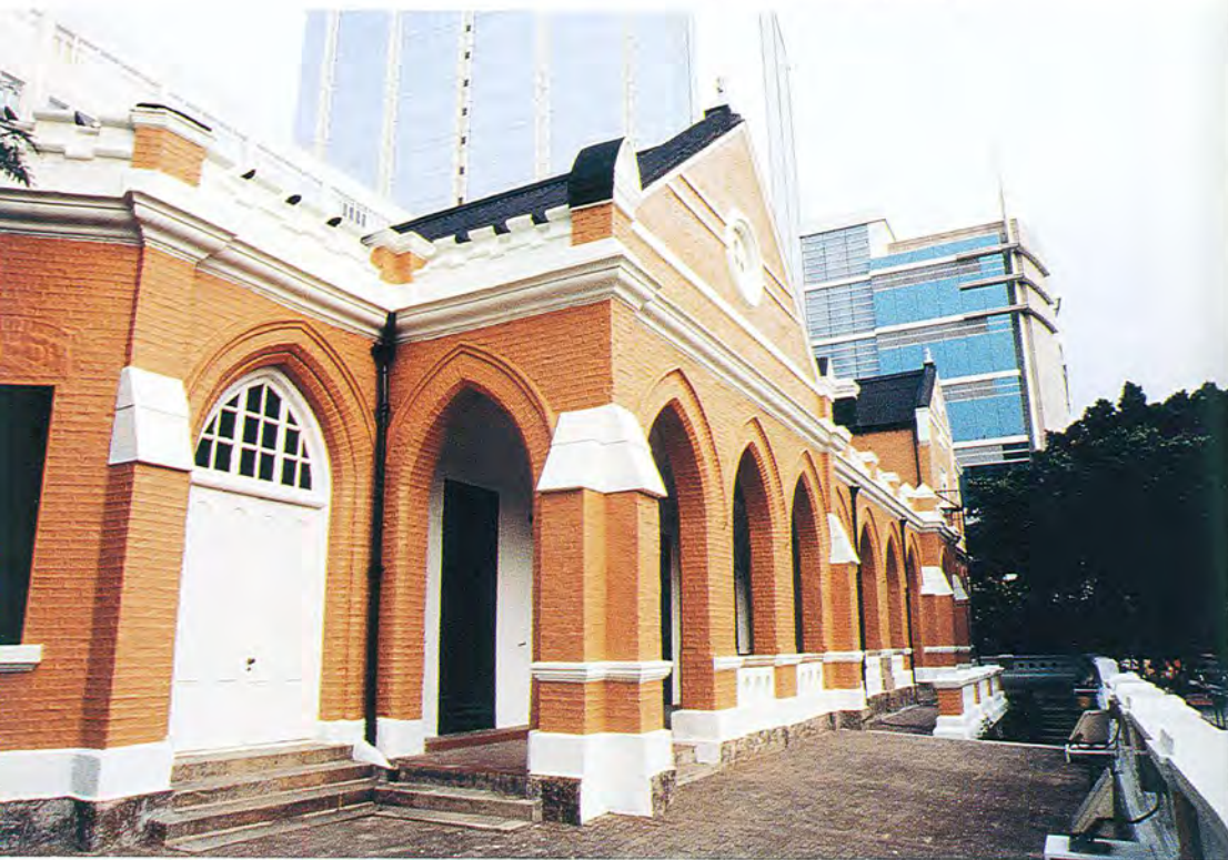
修繕後的前九龍英童學校 Former Kowloon British School after restoration.
