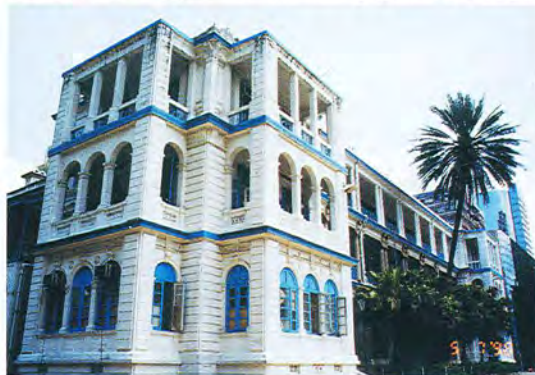
一九九八年的前水警總部 Former Marine Police Headquarters Compound, 1998.
