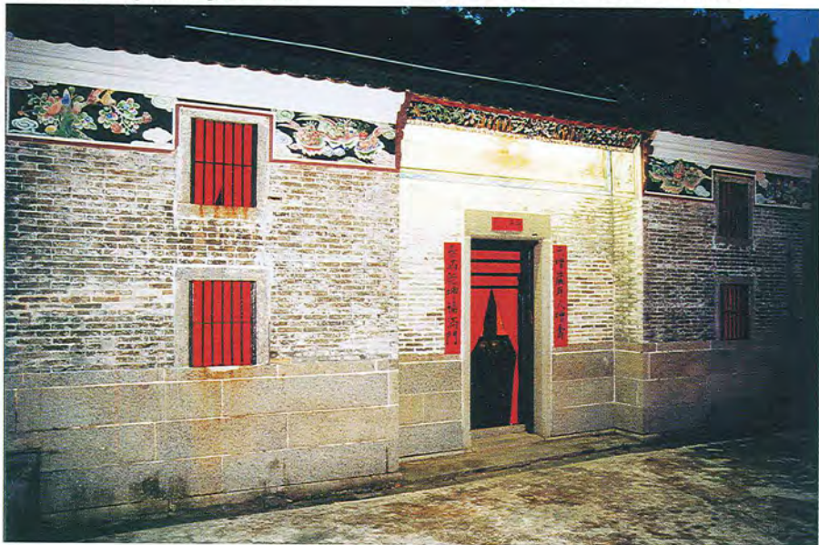
沙田王屋村古屋 Old House, Wong Uk Village, Sha Tin.
